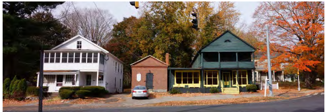
Empty commercial buildings along Woodbury's Main Street.
