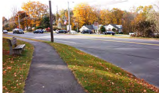
Typical asphalt on grade sidewalk.
