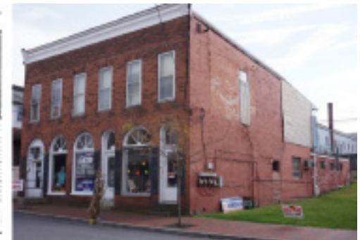
Vacant lot that could be used for outdoor dining in front and parking in back.
