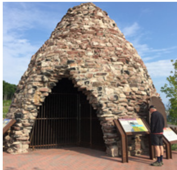
The Iron Ore Heritage Trail in Marquette Michigan provides a precedent of how a kiln can attract residents and visitors. The trail combines recreation with the story of a rich iron ore history-- in this case a beehive kiln used for making charcoal.
