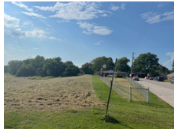
The Ohio River Greenway from start of the flood control levee at Greenmeadow to the end of the levee at 1st Street is an easy first step.
