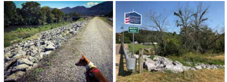
Views along the river walk atop the Army Corps of Engineers levees
