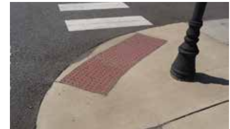
Traffic light pole in front of curb ramp
