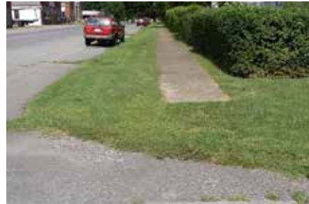
Walkway ends before connecting to street
