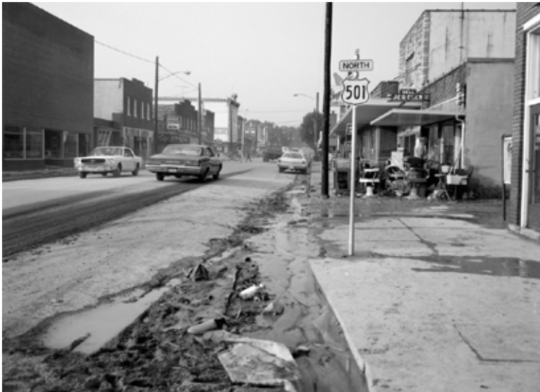
Magnolia Street in Buena Vista after Hurricane Camille
