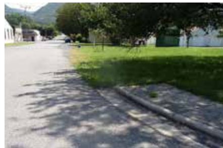
Walkway terminates at side street
