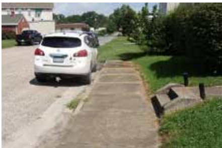
Walkway terminates mid-block
