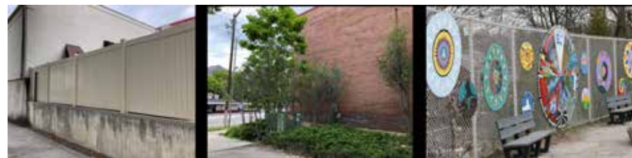
Successful screening, like at a loading dock or electrical transformer location (left, center) help reduce the visual impact of these service areas bringing a pleasant and orderly appearance to the street. Fences and screening can also be used to promote art and mural projects (right)
