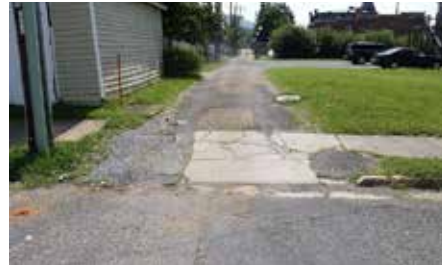
Alley entrances in poor condition with busted concrete, loose gravel and holes with standing water
