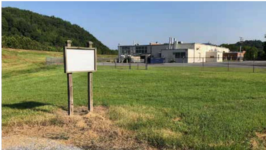
Existing River Walk parking lot and signage with the planned Agriculture Center (Mundet Factory) in the background - see enlarged plan for view location
