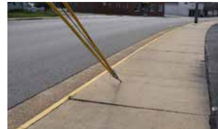
Utility pole cable in walkway
