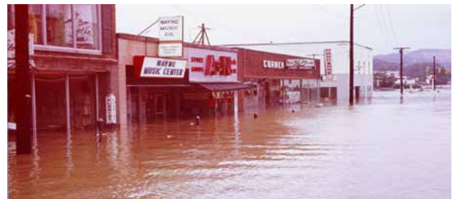
Shops submerged from the flooded Maury River
