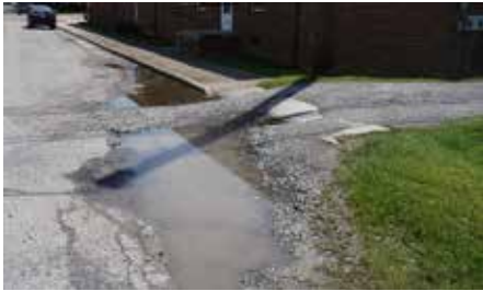
Alley entrances in poor condition with busted concrete, loose gravel and holes with standing water
