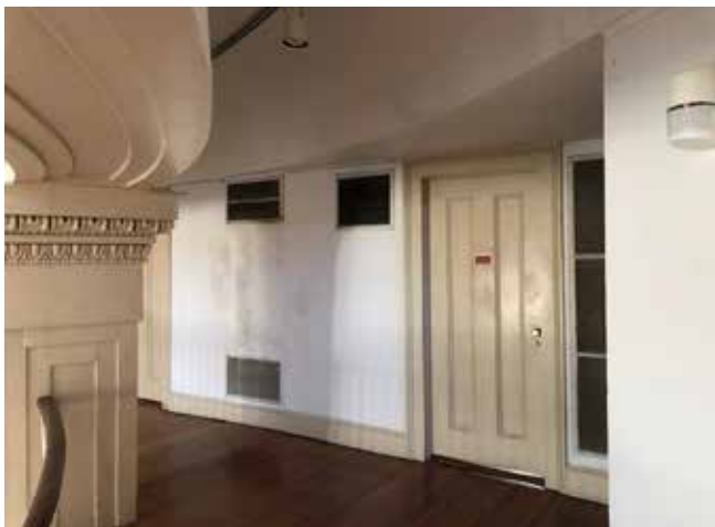
Views of moisture damage in the areas around mechanical grills and concealed ductwork around the Second Floor gallery.
