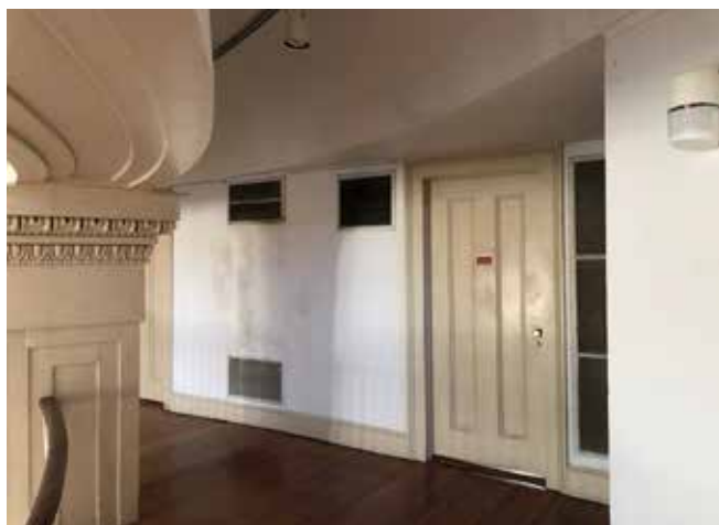
View on the Second Floor Corridor looking toward the door into Mechanical Room (201) showing mechanical grills in the corridor wall.
