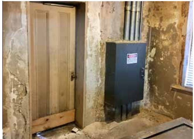
Ground water at the building's northeast corner has kept the walls wet and caused the deterioration of original plaster and masonry.
