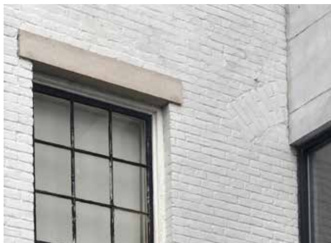
View of the small portion of brick segmental arch from original rear opening on the First Floor. Most of the arch is now hidden behind the elevator addition (right).
