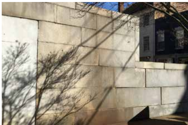
Views of the Front Portico west cheek wall with probable original infill in lighter stucco (Left) and granite steps detail showing settling and shifting (Right).
