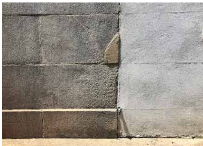
Detail at side of Front Portico where granite cheek walls meet ashlar stucco treatment.
