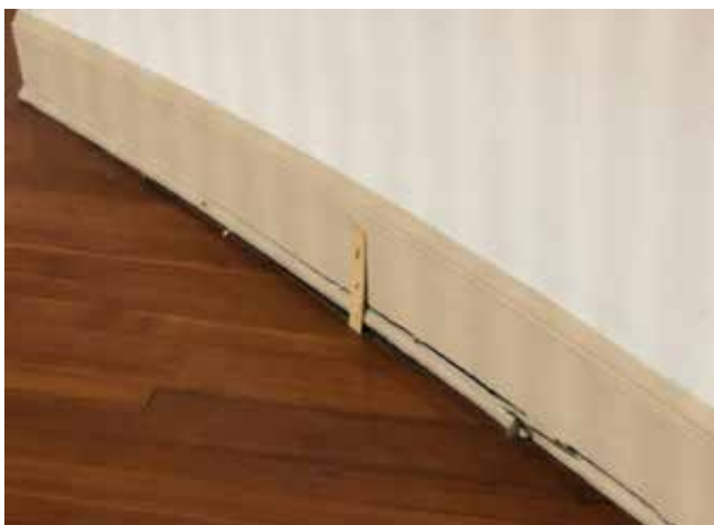
Southeast gallery location where floor has dropped and structural framing repairs are necessary (left), and moisture damage to arched plaster gallery ceiling (right).
