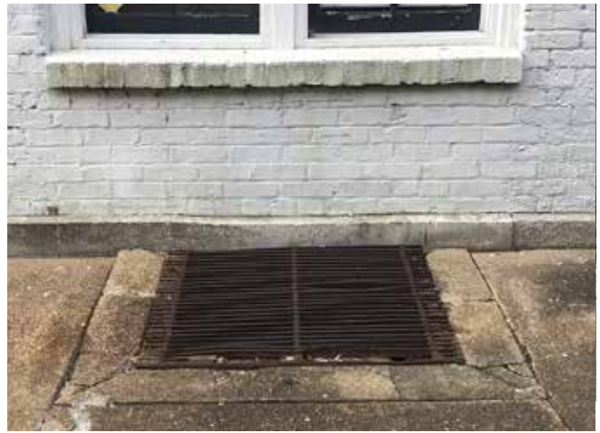
Coal chute (left), and surface grate (right) along the east alley side. A similar grated opening into the basement exists on the west alley side but has been filled in and paved over. With water flowing over the now low profile curb condition in the east alley, these openings are allowing a considerable amount of water into the basement which is migrating all the way to the center of the building
