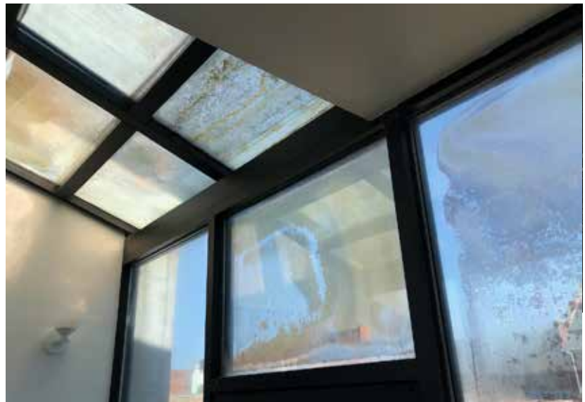
Interior views of the Second Floor of the elevator tower connector showing the condition of the glass and lack of integrated HVAC systems.
