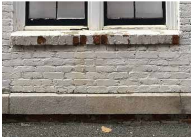
Shallow sloping threshold in the center indicates a center door at one time.
