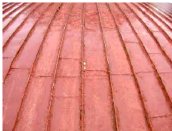
Detail of existing dome roofing showing segmented terne metal panels still intact.
