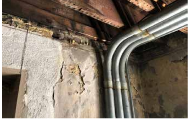
Views of interior plaster damage due to water infiltration (Left) along the west alley below the two story rotunda window and (Right) at the rear Ground Floor wall in the northeast mechanical room.
