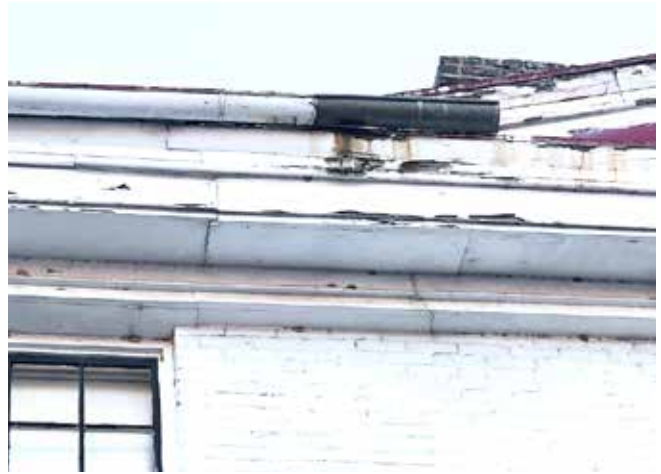
Symmetrical splices on both sides of the building's roofline with a stepped pattern most likely following the outline of the original cornice line from the portico as it extended out beyond the rear wall
