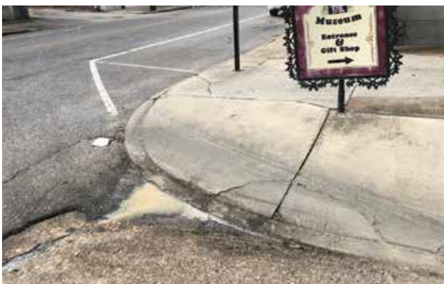
Views of the lowered curb at the southeast corner of the site (left) and showing the build up of paving along the east side alley curb allowing large amounts of water to flow over the curb towards the building. (right)
