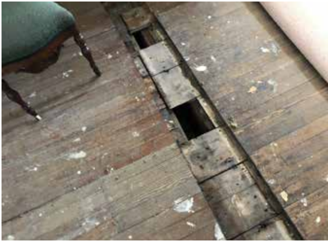
Detail in Meeting Room (203) showing evidence of two finish floor layers.
