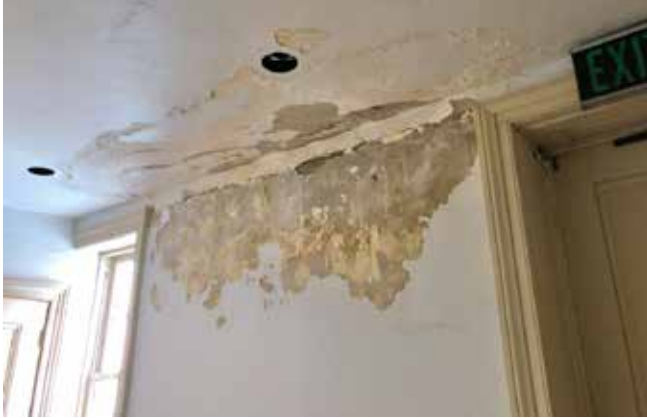
Views of interior plaster damage due to water infiltration (Left) along the west alley below the two story rotunda window and (Right) at the rear Ground Floor wall in the northeast mechanical room.
