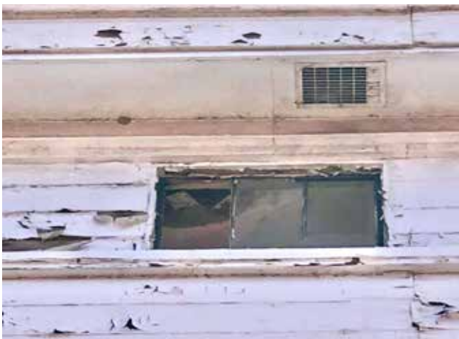
Views of cornice and frieze areas showing deferred maintenance and need for repair along with broken window panes.
