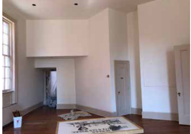
Gallery (104) showing 1970's build-outs for mechanical ducting — door to Stair (105) in center, door to Entry Hall (102) at right.
