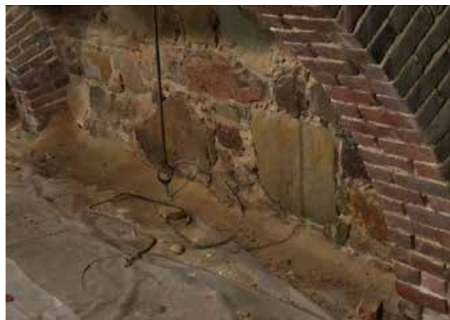
Basement views showing temporary 4x4 supports (left) and powdering mortar from both the stone and brick wall areas (right).
