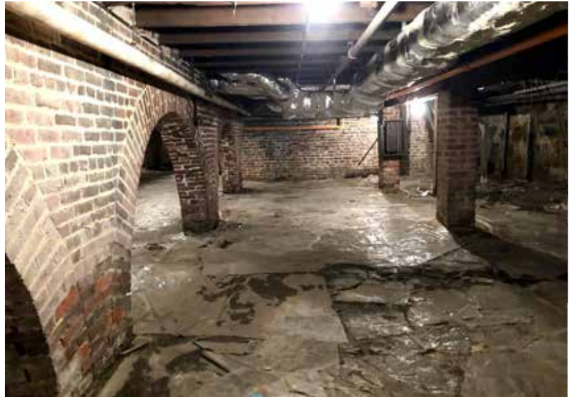
(left) view of the west alley opening infill showing that the window sash may have been installed to allow light into the basement near the stair location. (right) Basement view looking down center bay showing how water from the east alley grated opening has migrated (dark areas on floor) all the way to the center of the building
