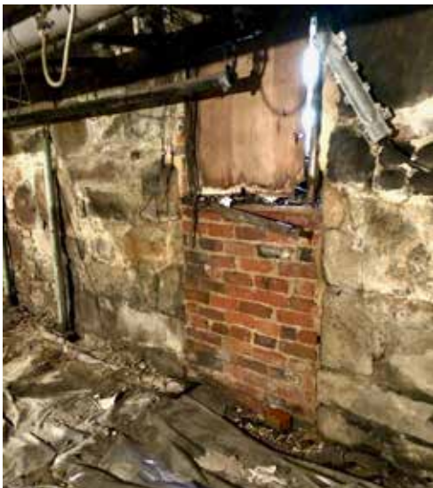
Interior Basement views of the bricked up, grated opening on the east alley where a considerable amount of water is coming into the basement.
