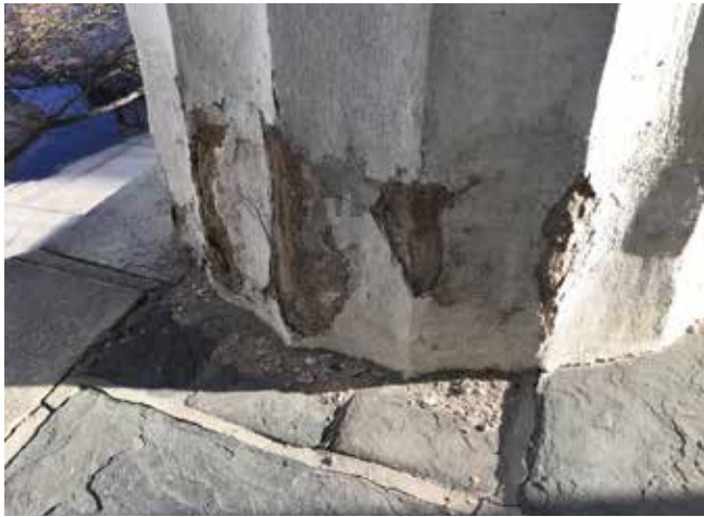
Views of flagstone floor and stucco on brick Doric columns showing deteriorated finishes..
