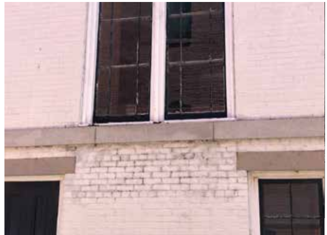
Water damage at exterior walls from splashing and damaged/rotted window sills and jamb members allowing water to get inside of the masonry walls and keep areas wet.
