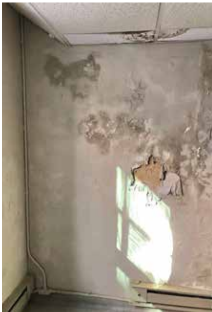
Interior views of plaster damage from sustained wall dampness.
