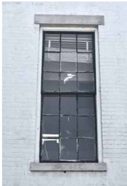
Typical exterior window views showing glazing that is falling out, broken panes and damaged sashes and sills.
