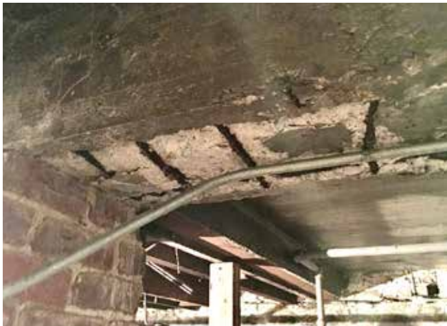
Basement moisture has caused spalling of structural concrete exposing and causing the deterioration of reinforcing steel.
