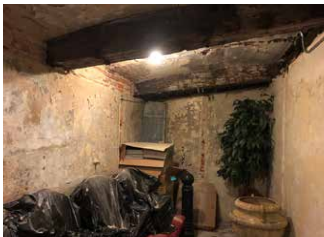
View into Foyer G-19 showing original plaster, beams supporting the portico floor above, and evidence of brick partitions.
