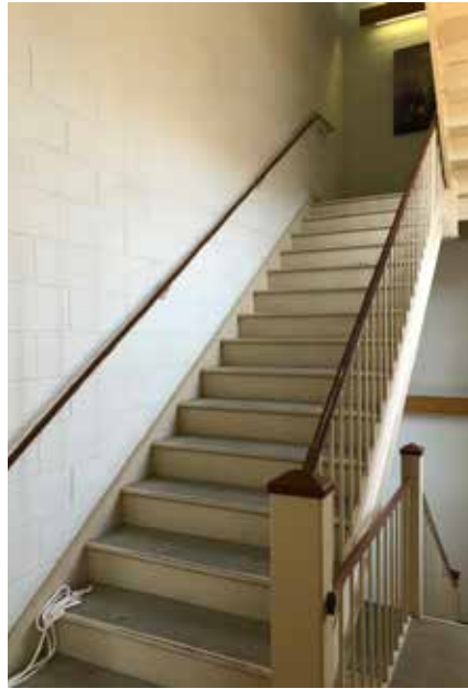
View from First Floor to Second Floor of 1970's Stair (122) with steel and concrete stair.
