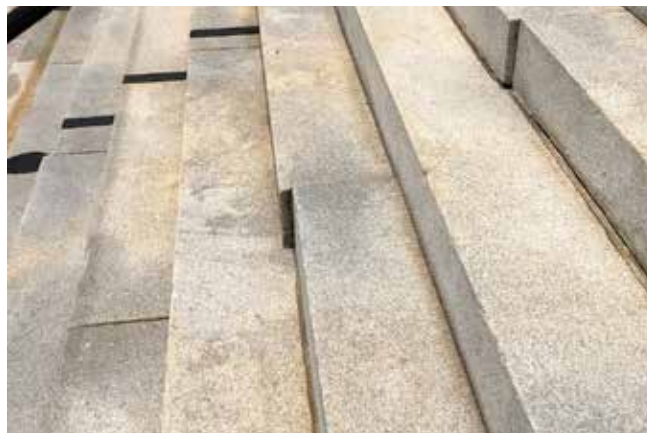
Views of the Front Portico west cheek wall with probable original infill in lighter stucco (Left) and granite steps detail showing settling and shifting (Right).
