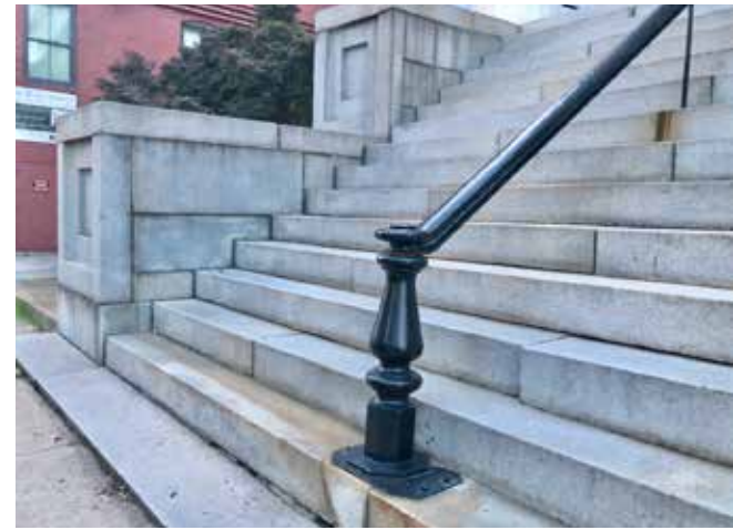
Shifting granite facing stones (left), and cast iron newel and railing with granite patch at mounting (right).
