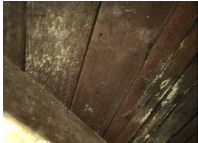
View of the entrance to the boiler room in the northeast corner of the Basement (left), and view of mold on Ground Floor joists and subfloor (right).
