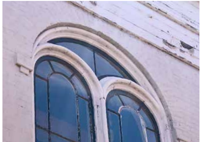
Detail at the top of the double arched window showing scalloped transom.
