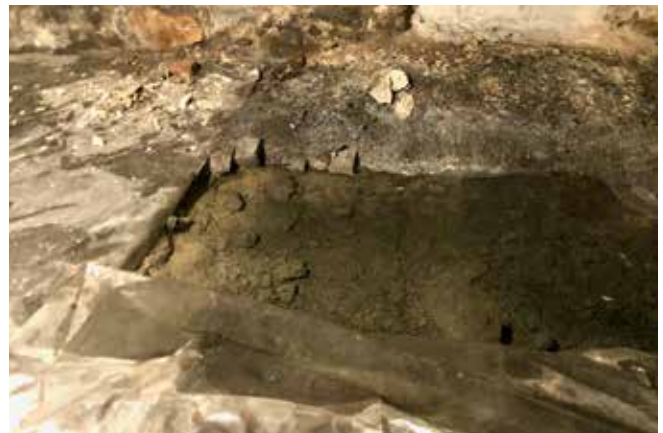
Views of the active water infiltration in the basement from ground water along the rear wall/parking lot. Standing water collects in low spots and fills up the Mechanical Room (two images below) when the sump pump is not working. The plastic on the ground in the basement helps with vapor but is installed over a build up of dirt that has accumulated on top of the original brick floor.
