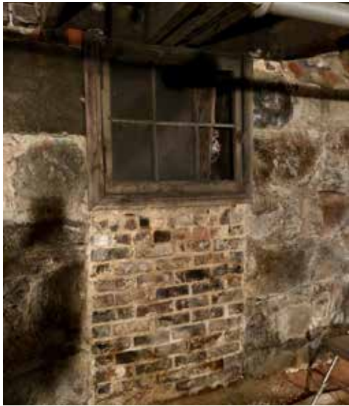
(left) view of the west alley opening infill showing that the window sash may have been installed to allow light into the basement near the stair location. (right) Basement view looking down center bay showing how water from the east alley grated opening has migrated (dark areas on floor) all the way to the center of the building
