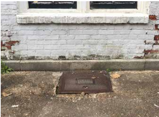
Coal chute (left), and surface grate (right) along the east alley side. A similar grated opening into the basement exists on the west alley side but has been filled in and paved over. With water flowing over the now low profile curb condition in the east alley, these openings are allowing a considerable amount of water into the basement which is migrating all the way to the center of the building
