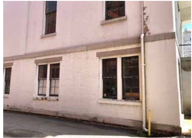
Views of existing gutters and poorly planned downspouts with leaking elbows and joints causing mortar and brick damage.
