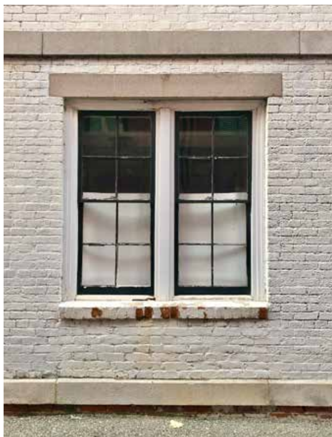
Most of the original alley openings have been filled in with 20th c. windows with brick sills.
