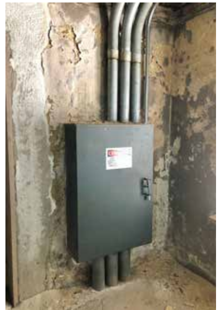
Views of interior plaster damage due to water infiltration (Left) along the west alley below the two story rotunda window and (Right) at the rear Ground Floor wall in the northeast mechanical room.
