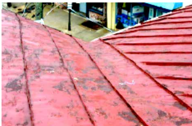
Detail of existing roofing showing long panels and oil-canning along with severe rusting
