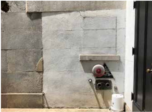
Fire department connection at the east side of the Front Portico (left), and Mechanical/Electrical Room on Ground Floor (right).
