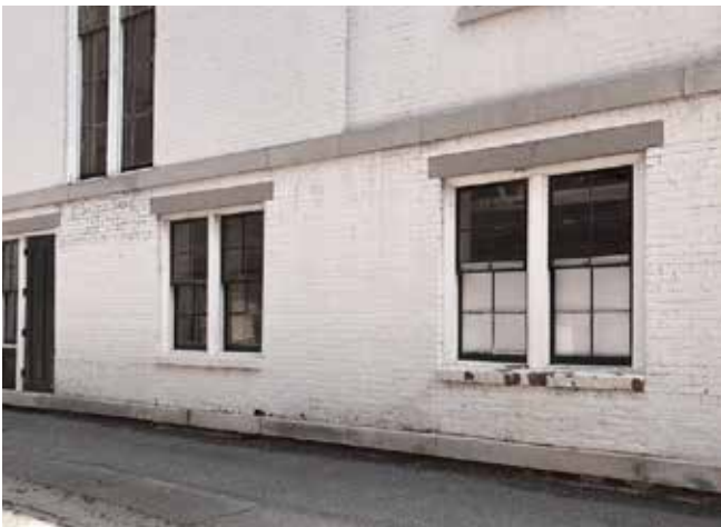
View of 4-over-4 window infills with brick sills at alley openings. Typical of both alley sides.
