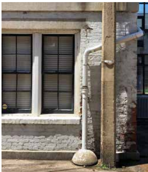
Masonry damage from walls staying moist due to water dripping from leaks in the gutter system above and splashing on the concrete walk at grade.
