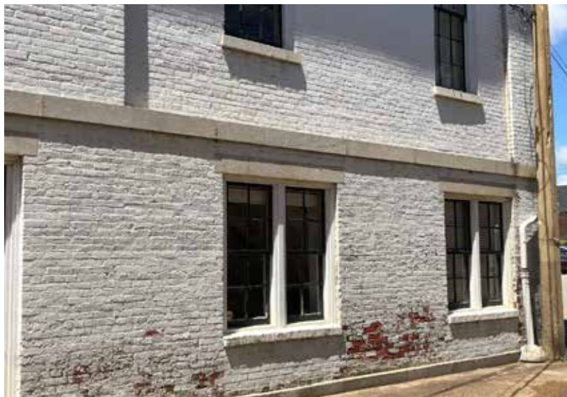
Masonry damage from walls staying moist due to water dripping from leaks in the gutter system above and splashing on the concrete walk at grade.
