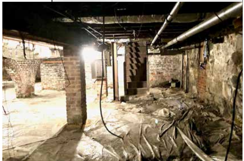
Interior Basement views of the bricked up, grated opening on the east alley where a considerable amount of water is coming into the basement.
