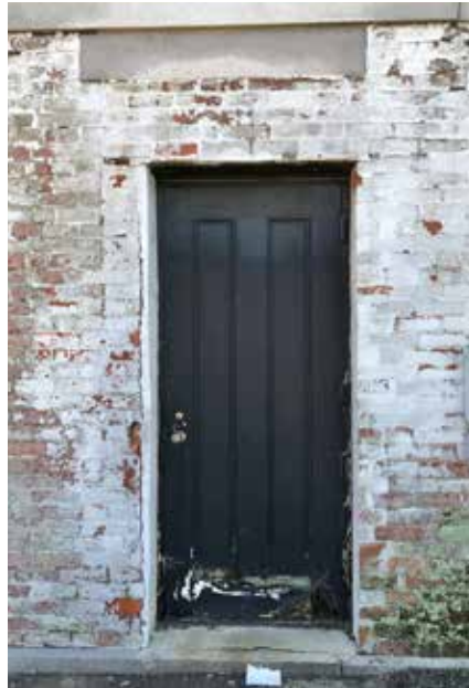
Image of condition of tall arched windows (left), Historic window infilled with door (center), Historic window infilled with louvers (right)
