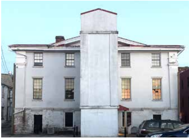
Evidence for the extent and location of the rear portico is clearly visible in the breaks at the First Floor belt course/window lintels as well as in the patching of the cornice and soffit where the portico roof was cut back
