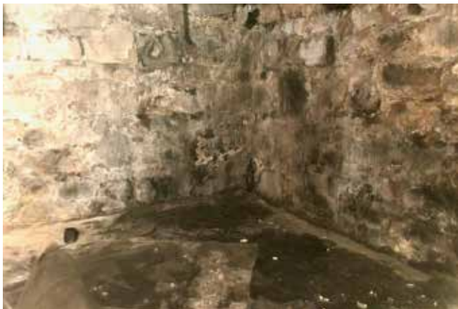
Views of the active water infiltration in the basement from ground water along the rear wall/parking lot. Standing water collects in low spots and fills up the Mechanical Room (two images below) when the sump pump is not working. The plastic on the ground in the basement helps with vapor but is installed over a build up of dirt that has accumulated on top of the original brick floor.
