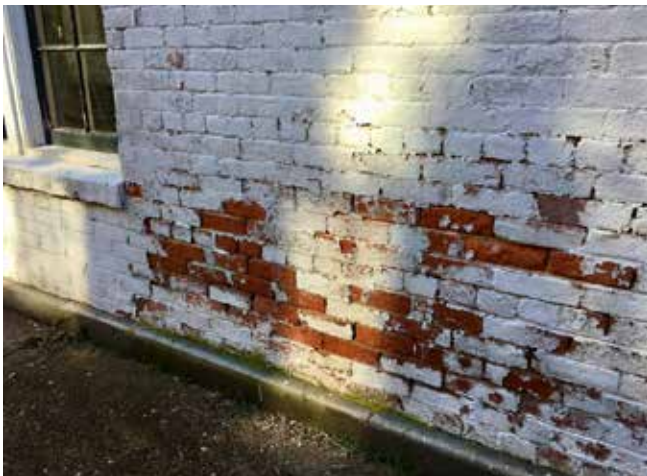
Water damage at exterior walls from splashing and damaged/rotted window sills and jamb members allowing water to get inside of the masonry walls and keep areas wet.
