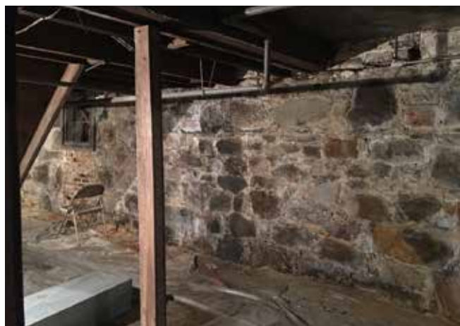
Basement views showing temporary 4x4 supports (left) and powdering mortar from both the stone and brick wall areas (right).
