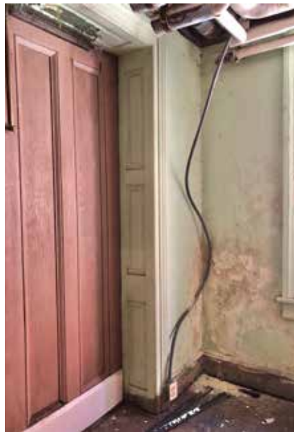
Views of interior plaster damage due to water infiltration (Left) along the west alley below the two story rotunda window and (Right) at the rear Ground Floor wall in the northeast mechanical room.
