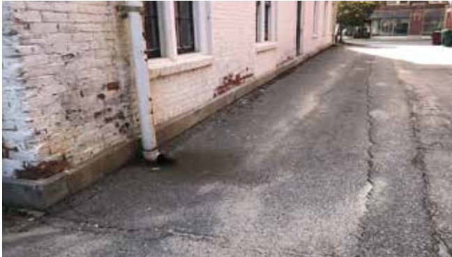
West alley views from back to front showing brick damage from water splashing on the pavement at the building wall as well as how paving, over time, has raised the alley surface up higher than the downspout outlet.
