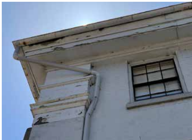
Existing exterior hung half-round gutters and downspouts.
