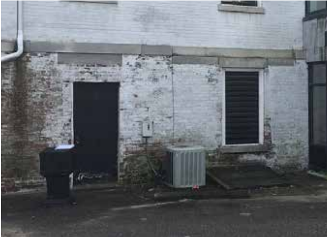
Water issues and deferred maintenance are causing deterioration of historic fabric.
