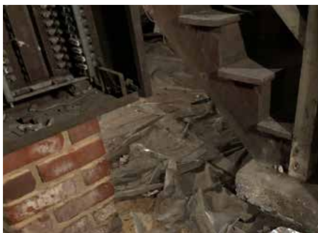
Basement views showing stairs from Ground Floor and brick piers deteriorating at their base.
