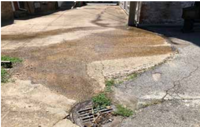
(left) Site drain behind the building in the east alley is insufficient to manage the amount of water draining from all of the paved areas around and behind the building. (right)
