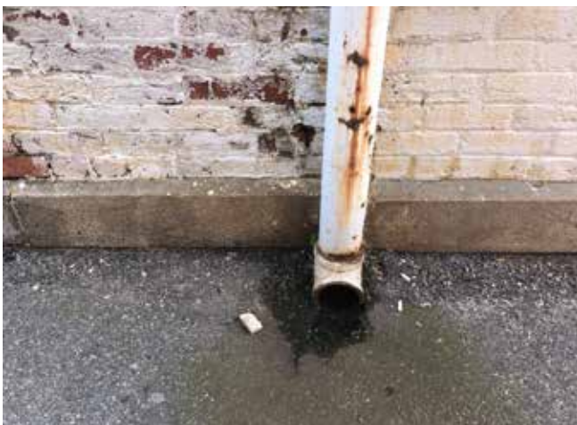
Views of existing gutters and poorly planned downspouts with leaking elbows and joints causing mortar and brick damage.
