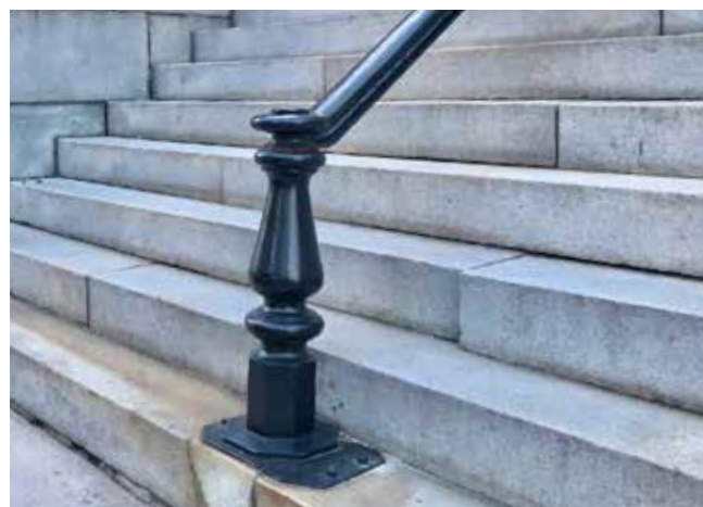
Detail of cast iron newel post at front steps
