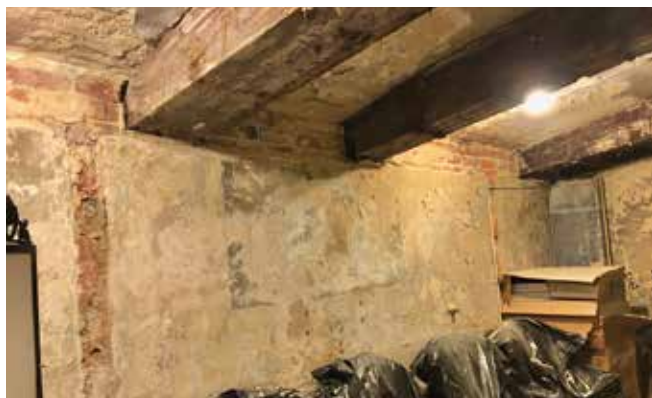
Views of the east room below the Front Portico showing curved wood beams and vaulted brick ceiling along with the remains of plaster finishes. The CMU infill of the original east doorway can be seen in the photo on the right.
