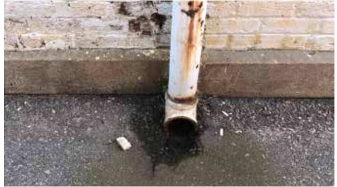
West alley views from back to front showing brick damage from water splashing on the pavement at the building wall as well as how paving, over time, has raised the alley surface up higher than the downspout outlet.
