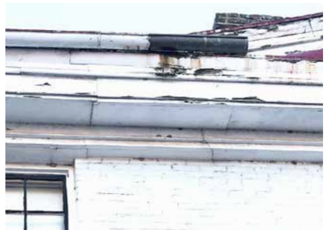
Stepped seams in the cornice and fascia where original rear portico pediment extension was removed and patched.
