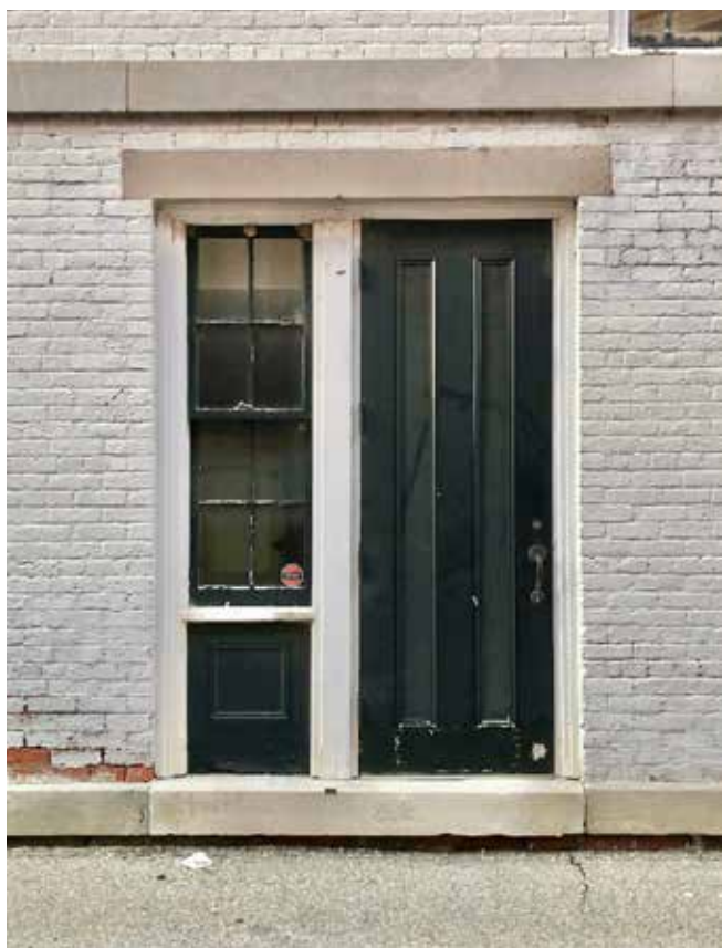
View of an original alley opening with a door and sidelight infill. Note the granite sill shows evidence of an earlier centered door.
