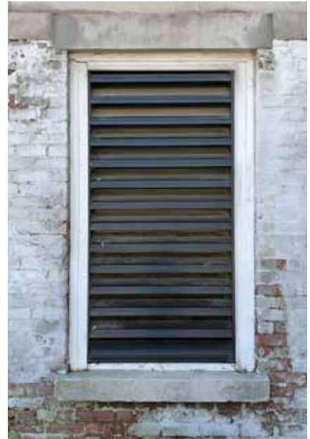
Image of condition of tall arched windows (left), Historic window infilled with door (center), Historic window infilled with louvers (right)
