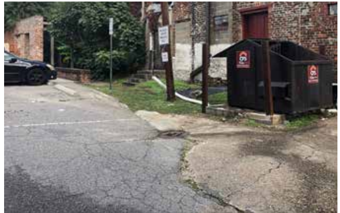
(left) Site drain behind the building in the east alley is insufficient to manage the amount of water draining from all of the paved areas around and behind the building. (right)
