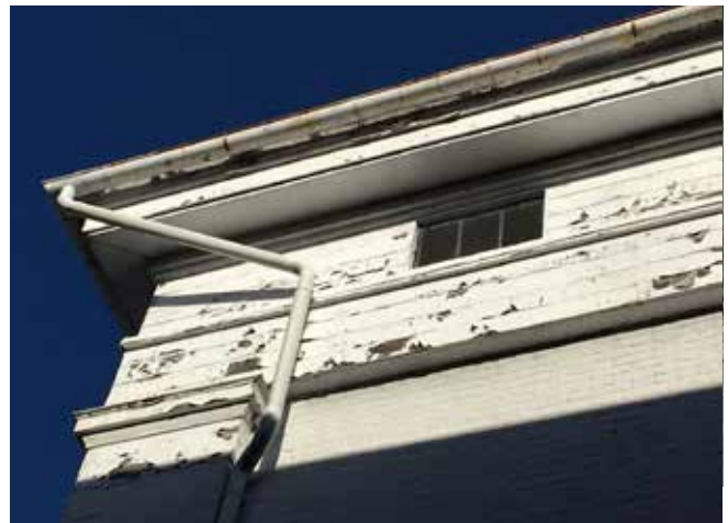
Views of cornice and frieze areas showing deferred maintenance and need for repair along with broken window panes.
