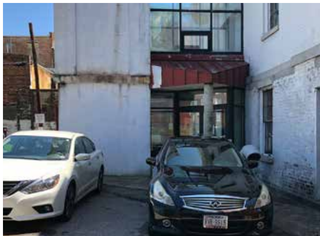
Rear entrance at the elevator tower showing the metal canopy and concrete sonotube column at the storefront system entrance doors.
