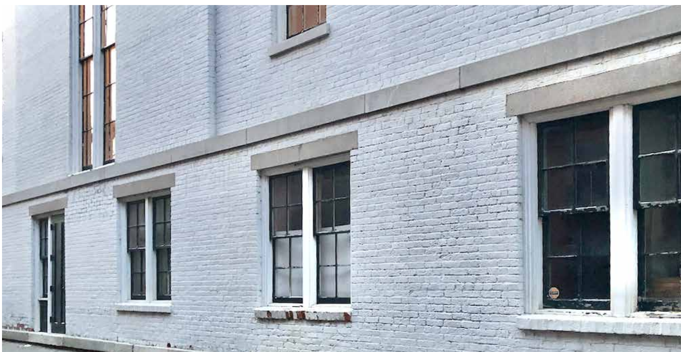
View down the east alley side (west is similar) showing original openings infilled with double windows and brick.
