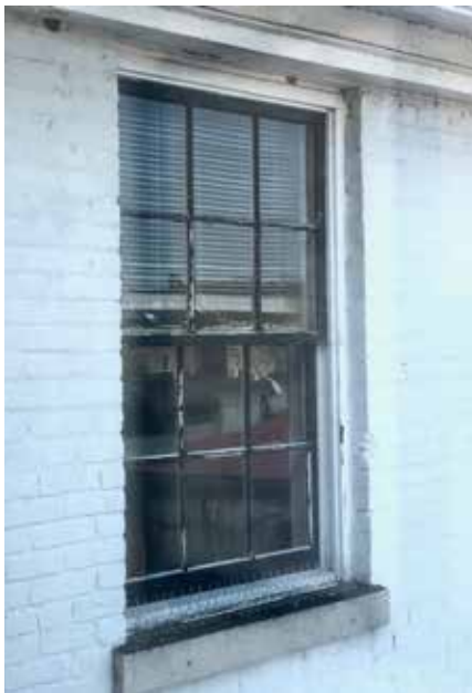
Typical exterior window views showing glazing that is falling out, broken panes and damaged sashes and sills.
