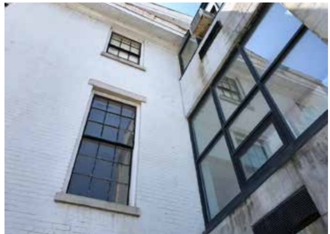
How the modern elevator tower meets the historic building.
