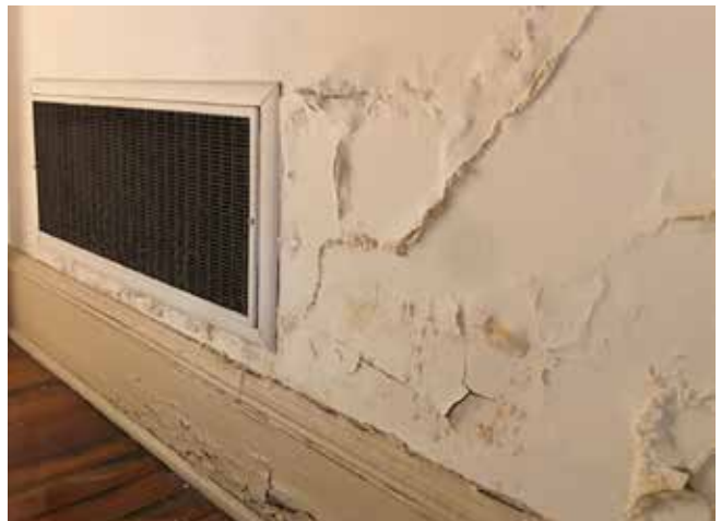
Views of moisture damage in the areas around mechanical grills and concealed ductwork around the Second Floor gallery.
