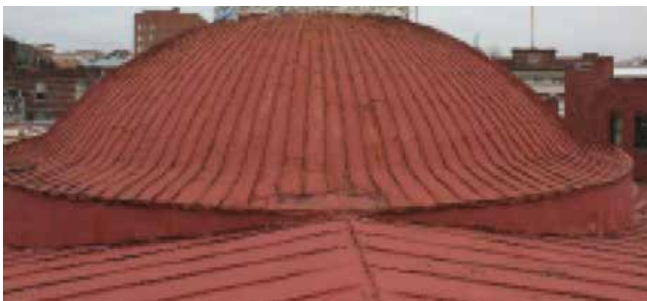
Close up of the dome showing its original soldered terne metal roof
