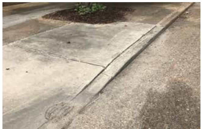
Views of the lowered curb at the southeast corner of the site (left) and showing the build up of paving along the east side alley curb allowing large amounts of water to flow over the curb towards the building. (right)
