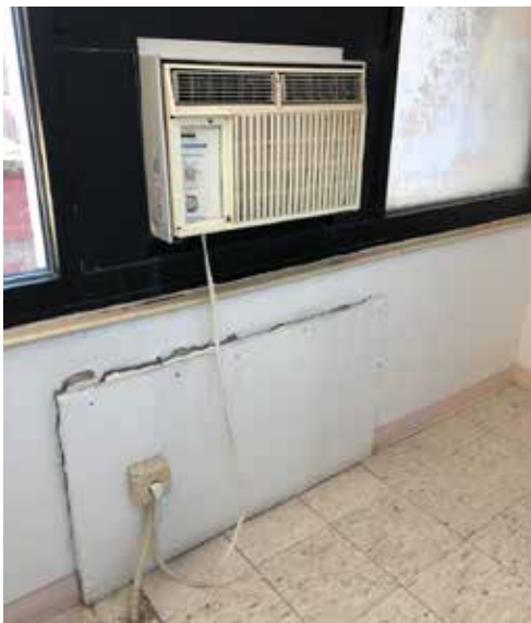
Interior views of the Second Floor of the elevator tower connector showing the condition of the glass and lack of integrated HVAC systems.
