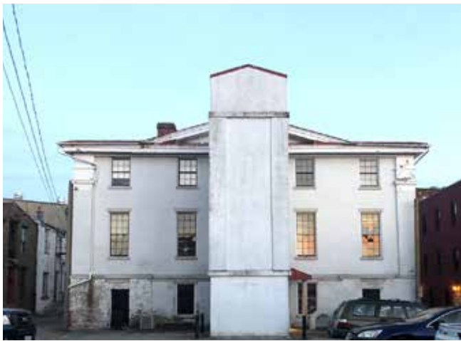
View of the rear or north building elevation showing 1970's elevator tower in the center and window pattern.
