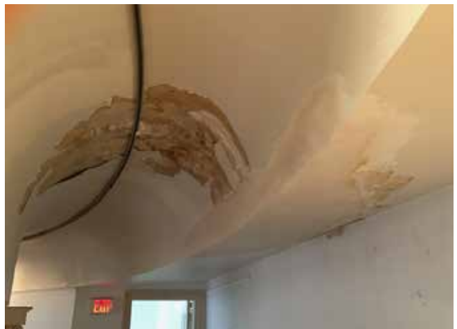
Southeast gallery location where floor has dropped and structural framing repairs are necessary (left), and moisture damage to arched plaster gallery ceiling (right).
