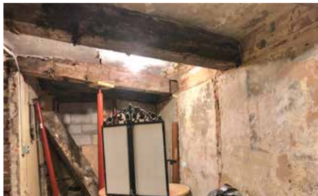
Views of the east room below the Front Portico showing curved wood beams and vaulted brick ceiling along with the remains of plaster finishes. The CMU infill of the original east doorway can be seen in the photo on the right.
