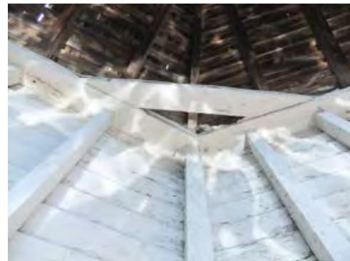
Figure 35: Top Plate Splice Detail
