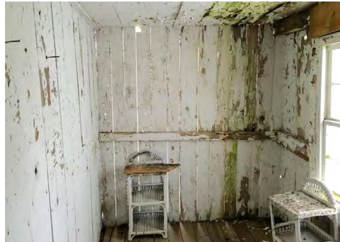
Fig. 112. Interior of East Wing looking north
