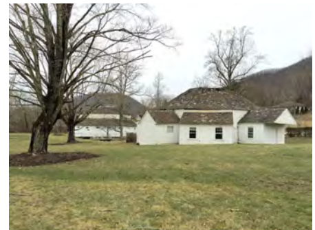
Fig 88. Octagonal Bath from northeast
