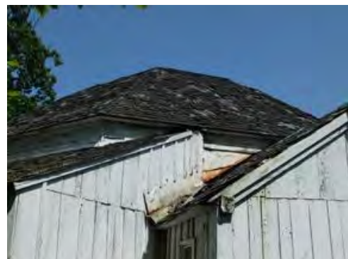
Figure 29: East Vestibule Flashing
