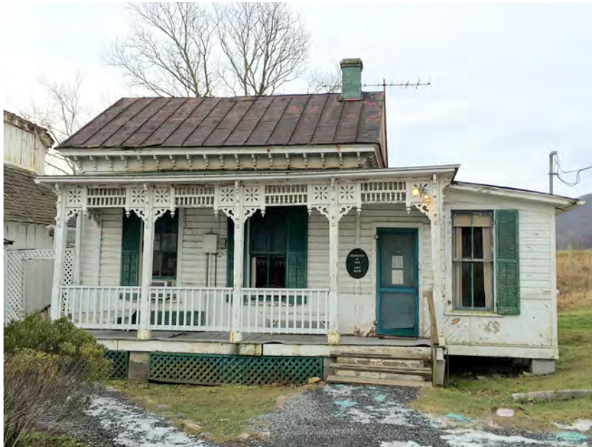
Fig. 131. Exterior of Reception House looking south.
