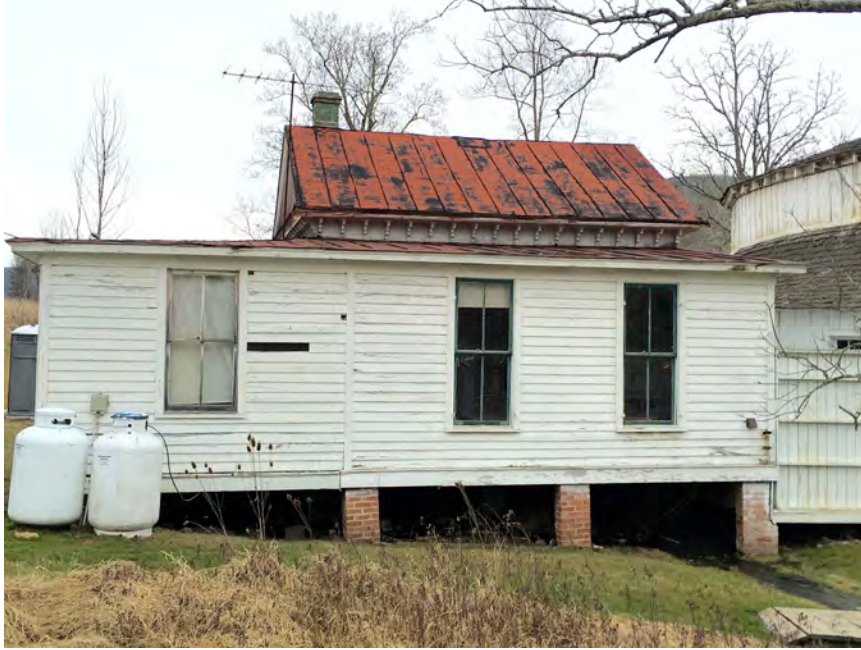
Fig. 132. Exterior of Reception House looking north.
