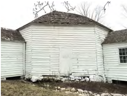
Fig 86. Southwest wall seen from southwest
