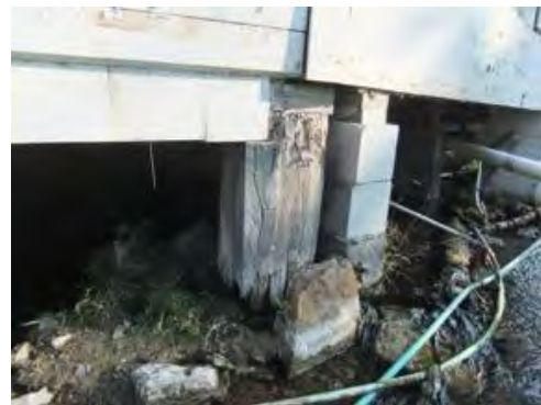
Figure 5: Timber Piles replaced with masonry piers
