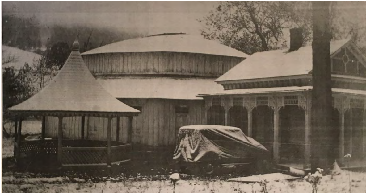
Fig. 71. The Ladies' Bath and Reception House in winter (1930s?). Collection of John T. Reddick. Note that the entry to the Drinking Spring is in the western bay. The parapet is missing
