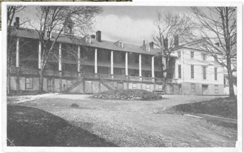
Fig. 18. c 1920 postcard of the Warm Springs Hotel, showing brick Main Hotel of the 1830s with the raised colonnade across the front and the added Dining Room wing of the 1850s to the right.
