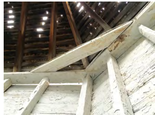
Fig. 90. Typical splice plate
