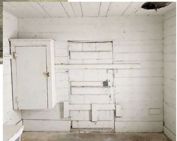
Fig. 103. Interior of North Wing looking north
