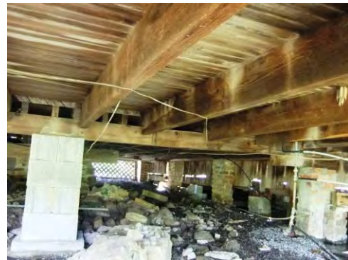
Figure 42: First Floor Framing
