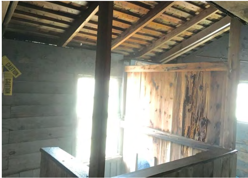
Fig 107. Spout bath leanto interior looking southeast
