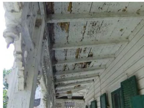
Figure 43: North Porch Roof Framing
