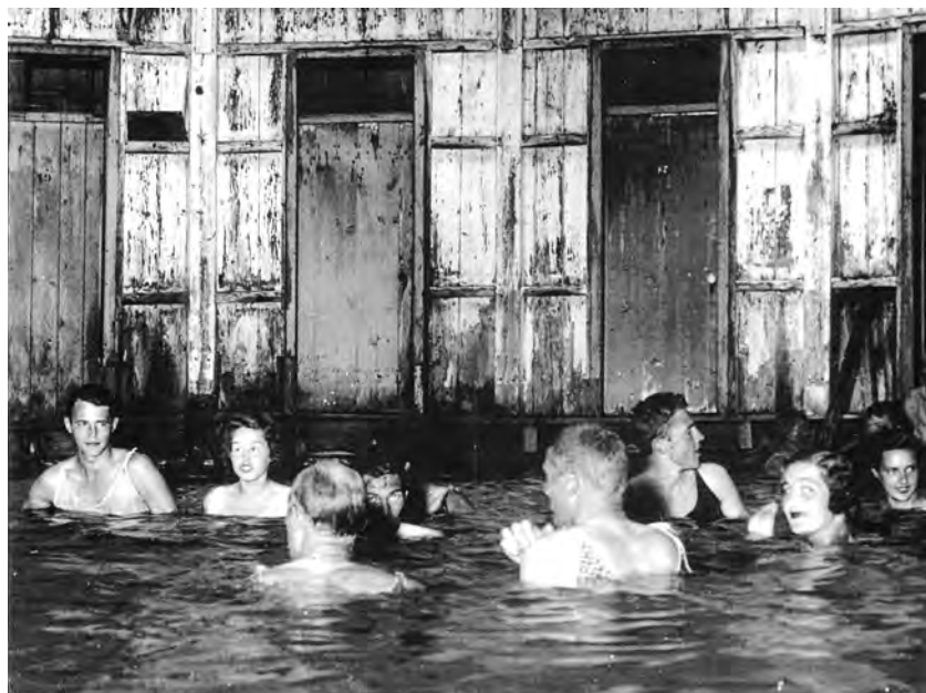
Fig 73. Ingalls family annual party at the Warm Springs in the Ladies' Pool, 1920s. Note the poor condition of the framing.
