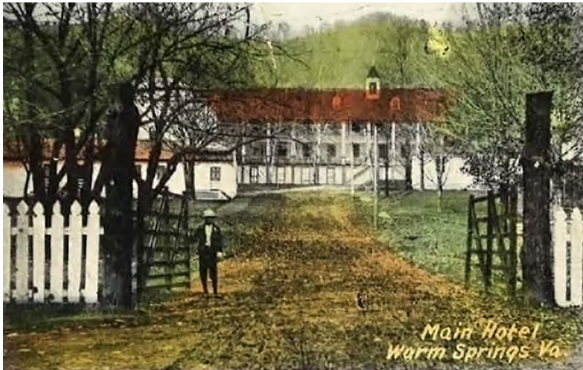
Fig. 32. Warm Springs. Early 20th-century postcard of the gate and flanking decorative fences at the entry to Warm Springs.
