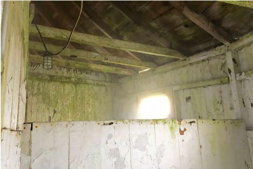
Fig 129. Original material in outer dressing room ring on the south side.
