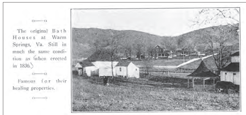
Fig. 44. Bath Buildings, 1930s (?), Bath County Historical Society. Note the claim that the bath houses were "built in 1836," fairly accurate for the octagonal bath. Also note the enclosed deck along the southwest side of the octagon, probably added in the 1930s.
