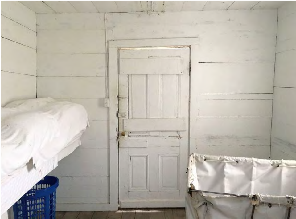
Fig 110. Interior of west wing from east
