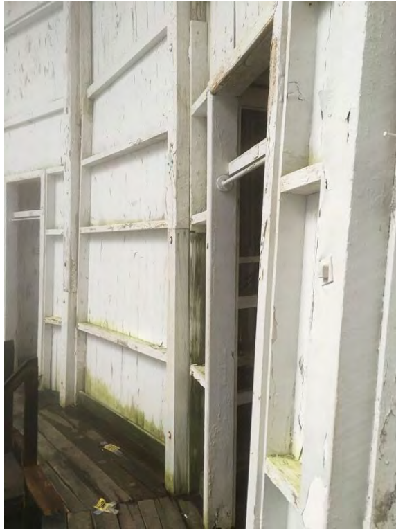
Fig. 124. Lower section of the interior wall (typical).
