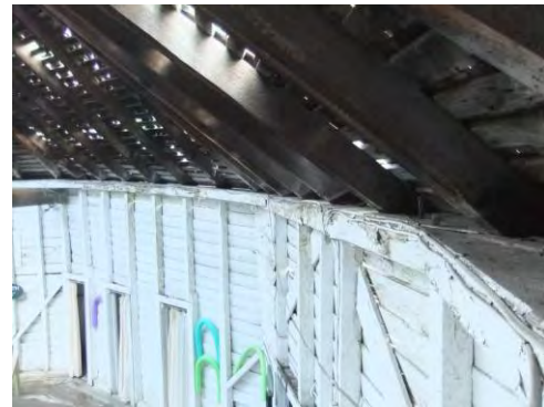
Figure 34: Top Plate Tension Ring
