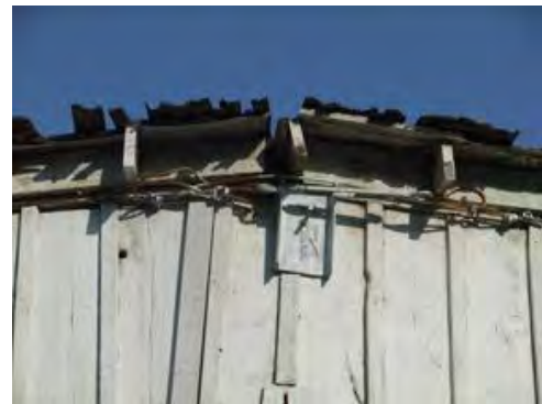
Figure 8: Retrofit cables and tie rods
