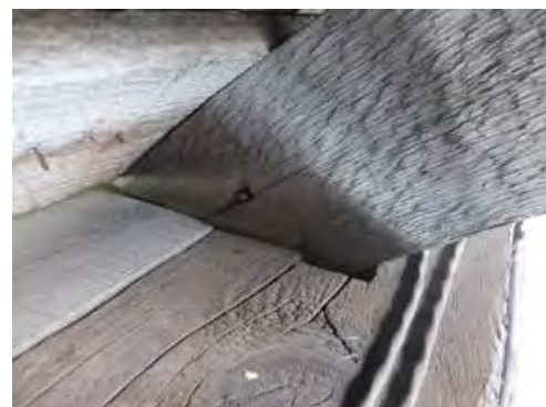
Figure 33: Top Plate Rafter Bearing
