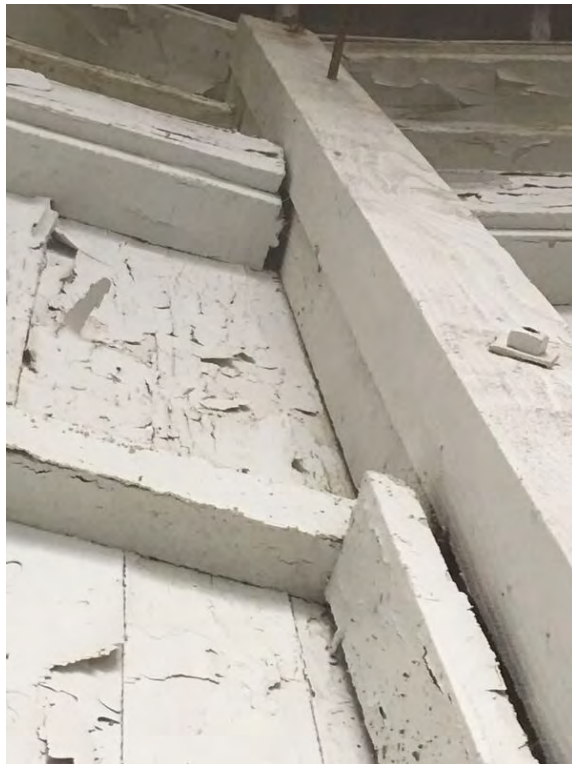
Fig. 125. View of typical inner ring wall showing mortise-and-tenon original upper structure and added face post and lower structure.
