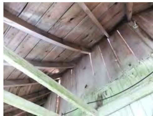
Figure 11: Curved rafters and framing at low perimeter roof.
