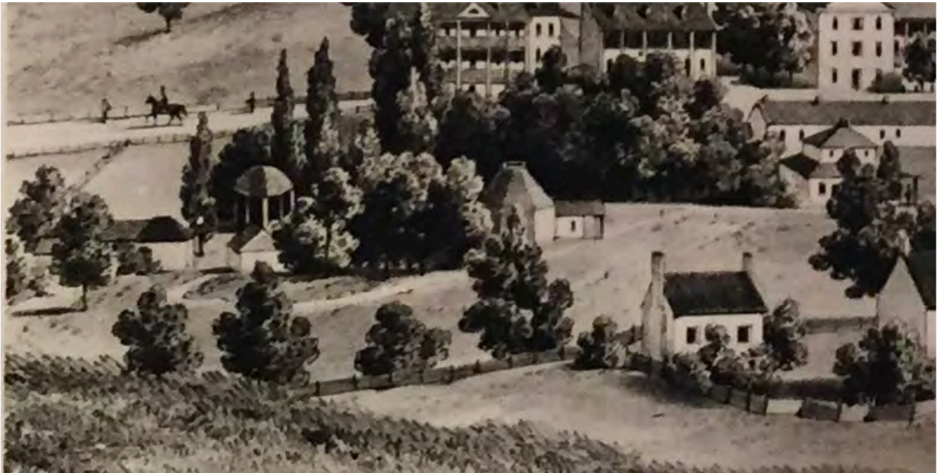
Fig. 53. Detail showing bath complex at the Warm Springs from Beyer's lithograph of 1850.
