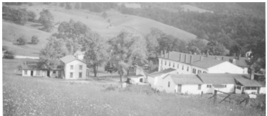
Fig 21. Warm Springs Hotel's north wing from the golf links to the northwest, no date. Library of Virginia.
