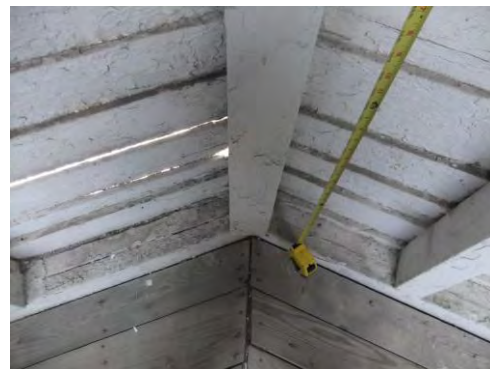
Figure 40a & 40b: Corner Post Plumbness
