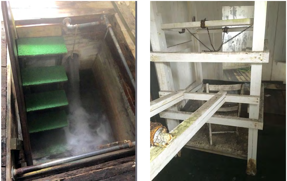
Fig 118. Brick tank for the spout bath on interior (left) and the rebuilt invalid lift (right)
