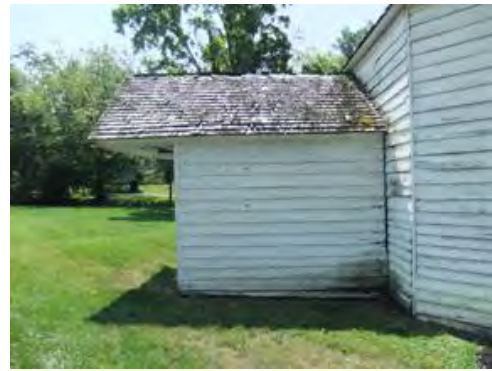
Figure 26: Entrance Vestibule - South
