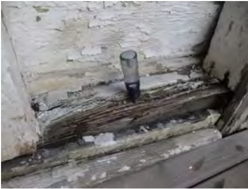
Figure 38: Sill Deterioration
