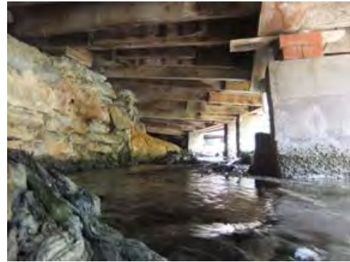
Figure 4: Foundations and Floor Framing
