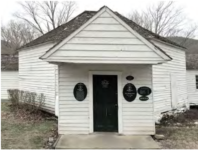
Fig 108. West wing from west.
