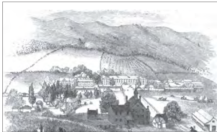
Fig. 22. Detail of Warm Springs by David Hunter Strother. Harper's New Monthly Magazine, vol. 10, no.57, Feb. 1855. Note the parapet around the oculus of the octagonal bath and the four dressing room wings, as well as the domed Drinking Spring and the small First Ladies' Bath. Note also the clump of trees next to the bath, probably the grove of elms mentioned by Mark Pencil in 1839. The drawing is so similar to Beyer's lithograph published in 1857 that it suggests that Porte Crayon's drawing was used as a model by Beyer. The building to the right of the bath is the Brockenbrough Cottage, used by the Robert E. Lee family after the Civil War.
