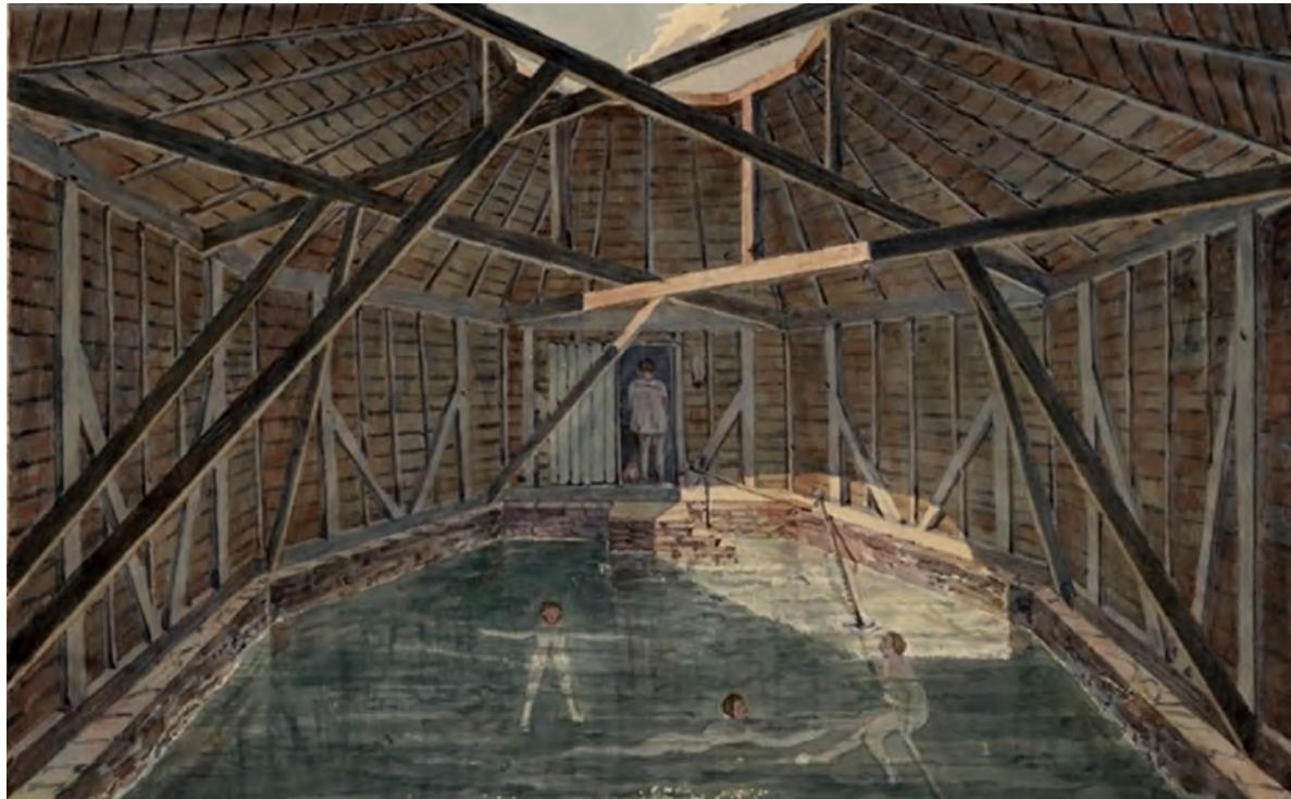
Fig. 38. J. H. B. Latrobe. Bath at Warm Springs [usually misidentified as the “Women’s Bathhouse”], 1832. Maryland Historical Society, Baltimore. Note the roof support structure and the projecting ledge of the stone basin wall, as well as the bathkeeper waiting in the door of the changing room.
