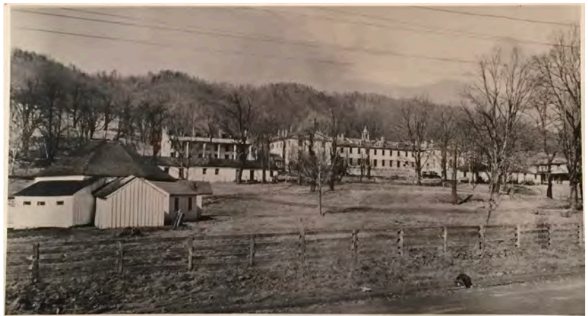
Fig. 59. Warm Springs, c. 1925. The hotel, which has lost its porch, appears to be under demolition. Note the stove chimney visible on the north dressing room roof and the lack of posts supporting its porch roof.
