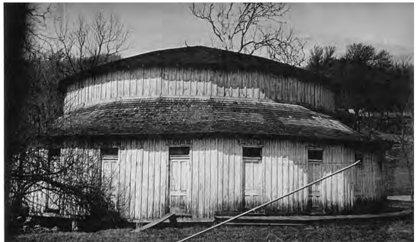
Fig 67. The Ladies' Bath in the mid-1930s. Historic American Building Survey, mid-1930s. Library of Virginia.
