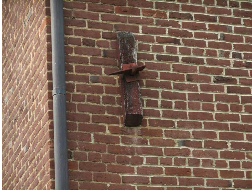
Figure 53: Tie rod anchorage at west end of south wall
