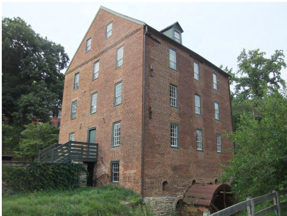
Figure 2: View of southwest corner of Waterford Mill
