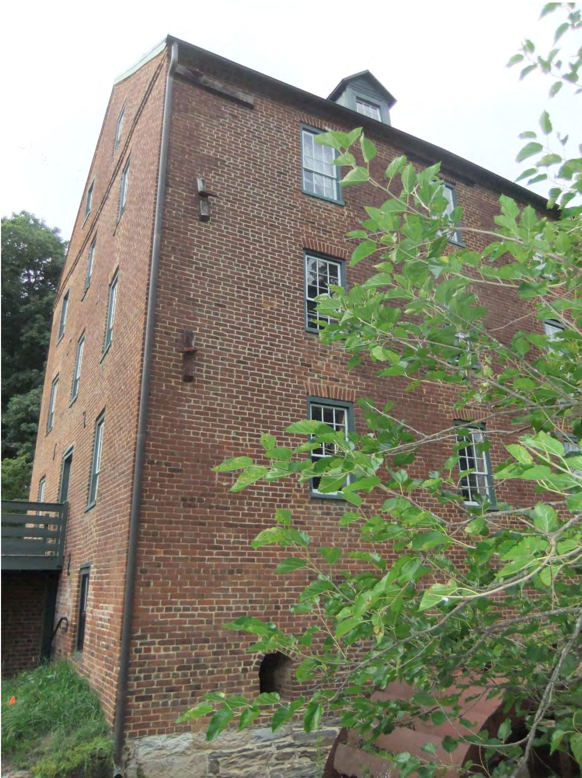
Figure 52: Tie rods at west end of south wall
