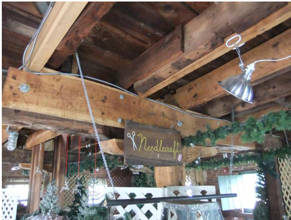
Figure 10: Attic level longitudinal beam sister reinforcement
