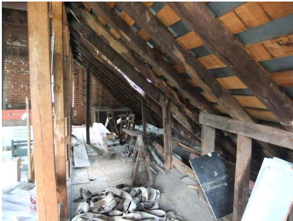
Figure 8: Intermediate support of rafters
