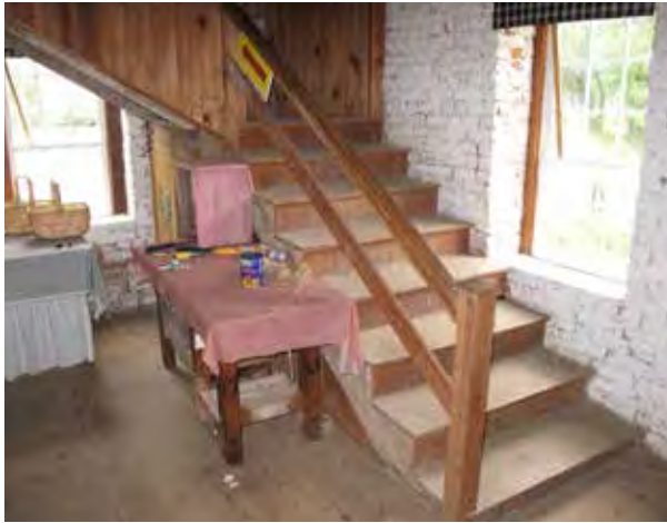
First-floor stair in southeast corner.
