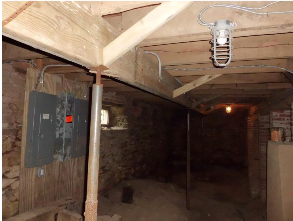
Figure 35: First floor shoring within northern joist bay
