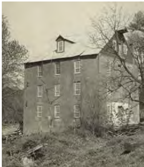
Waterford Mill soon after acquisition by Waterford Foundation in 1944 and after the west wing had been demolished. The corrugated metal roof appears loosely attached [WF].
