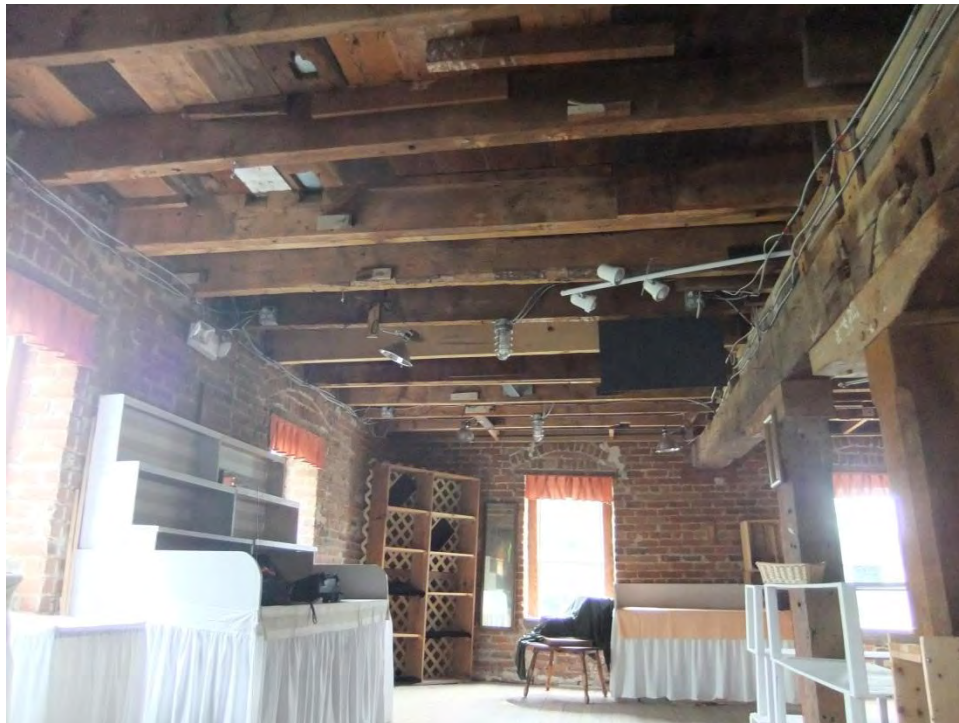
Figure 16: Third floor joists
