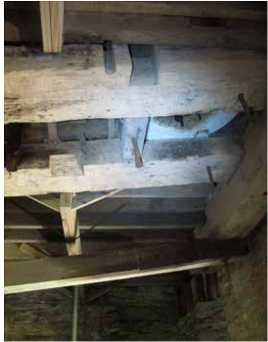
Right: Eastern millstones shifted to the south on original stone bearers.
