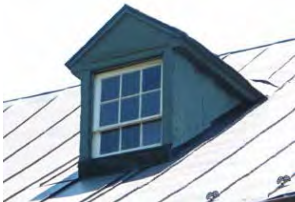
Close-up view of dormer
