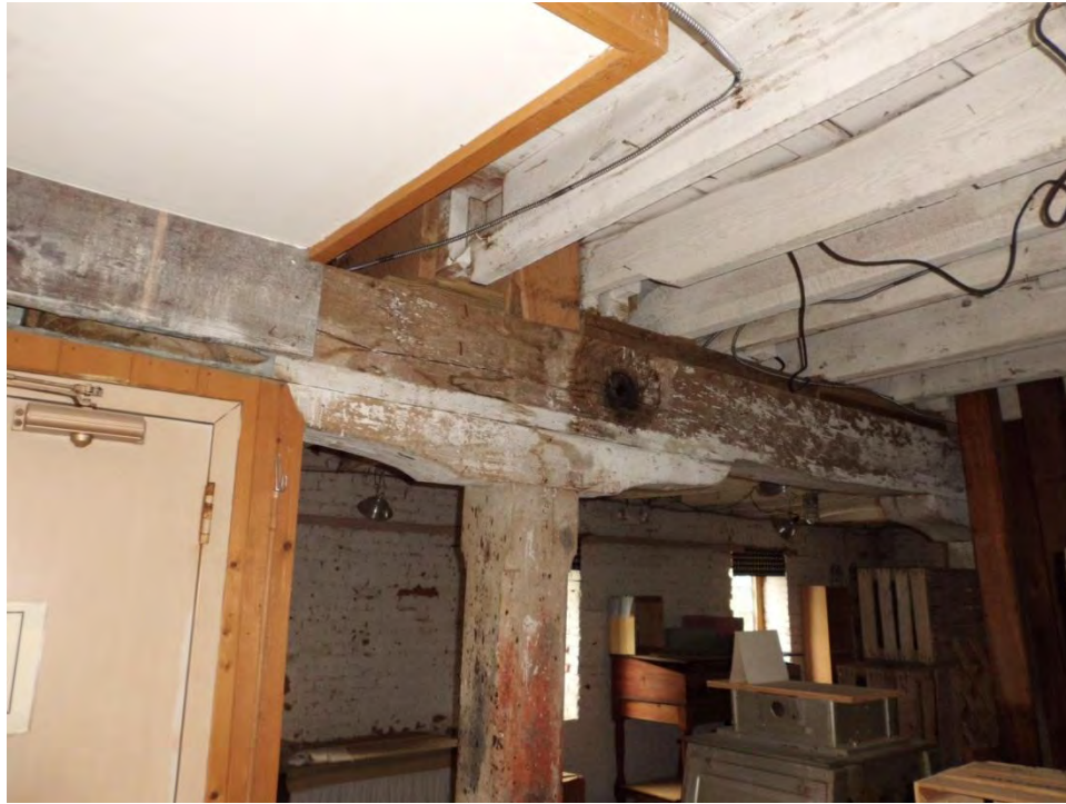
Figure 25: Second floor longitudinal beam notch
