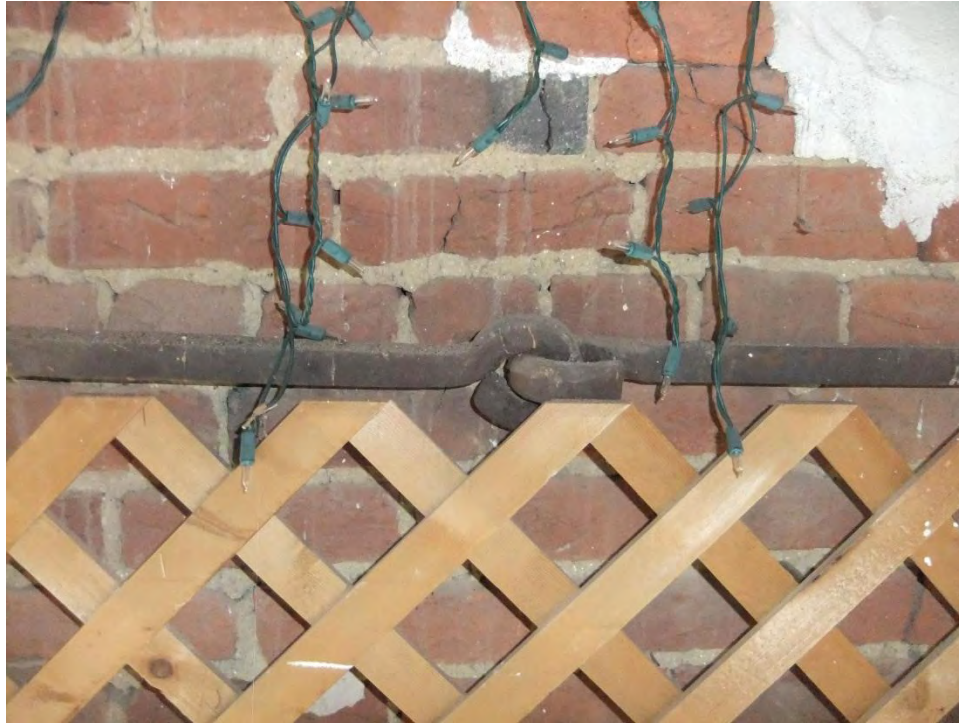
Figure 13: Attic level square tie rod connection
