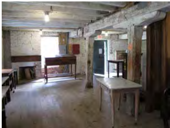
First floor looking east in north structural bay
