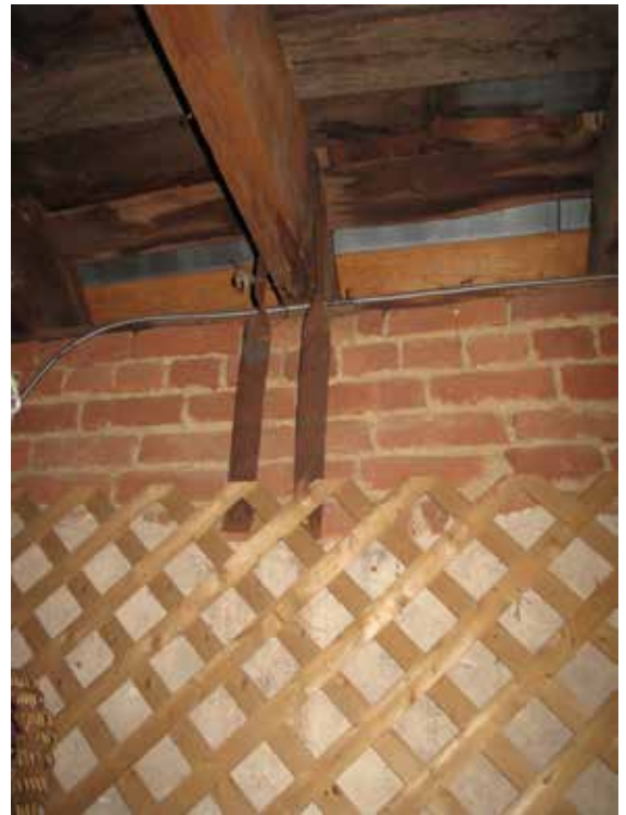
Typical metal strap along the third-floor north wall.
