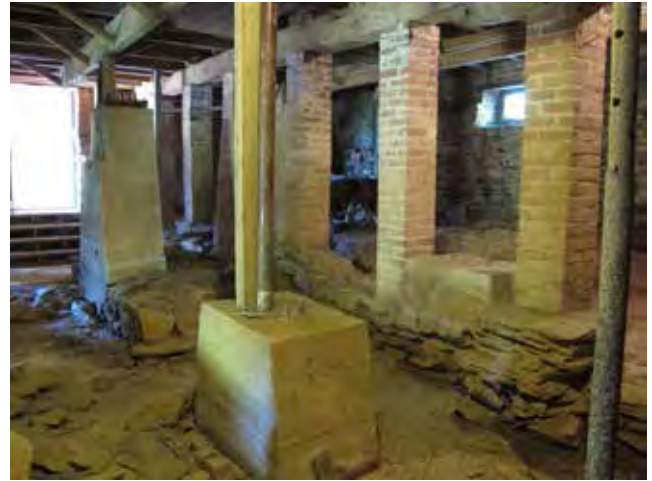
The central bay of the basement looking west.
