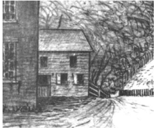
Detail of an 1882 sketch also shows a three-board fence running along the edge of the mill property [WF].
