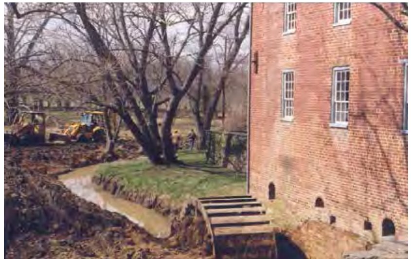
Waterford Mill, excavation of mill race, 1998 [WF].
