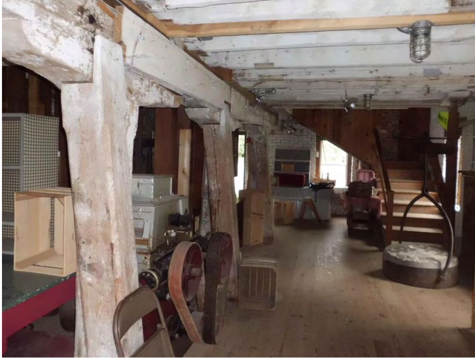
Figure 27: Second floor canted column brace
