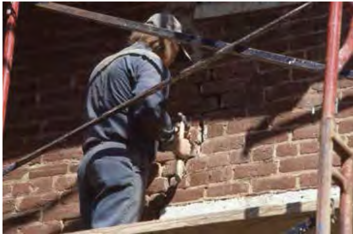
Removing portland cement repairs, south wall, April 1984 [WF slide collection]
