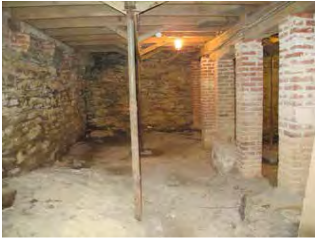
The north bay of the basement looking east
