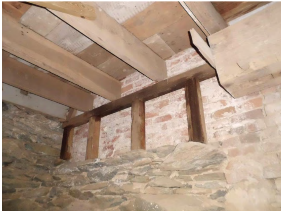
Figure 38: First floor southern joist wood knee wall
