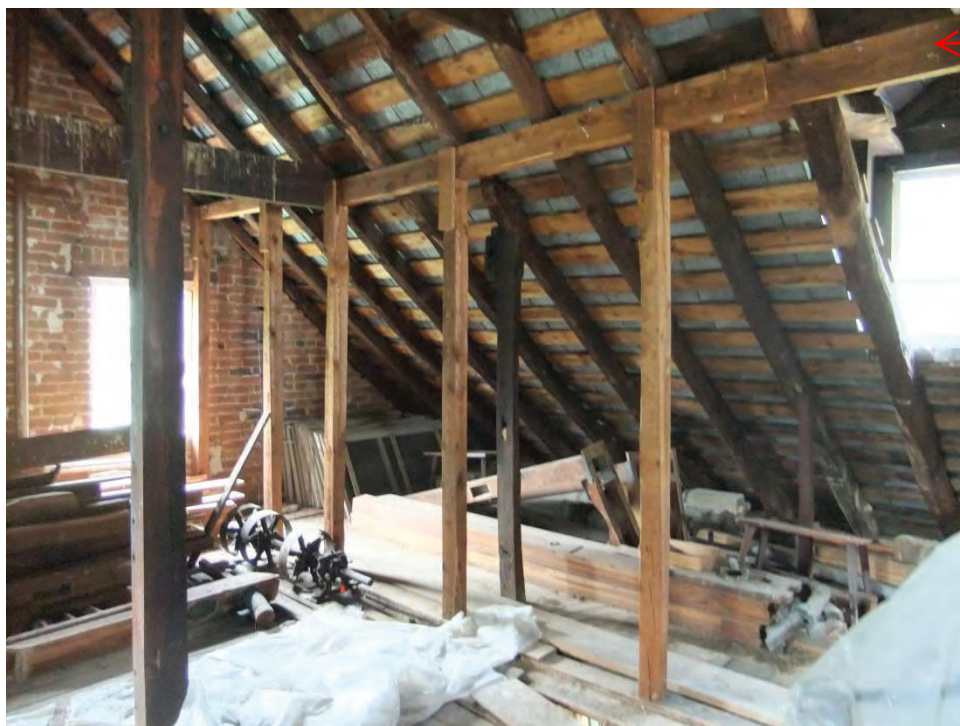
Figure 6: Roof purlin and post support
