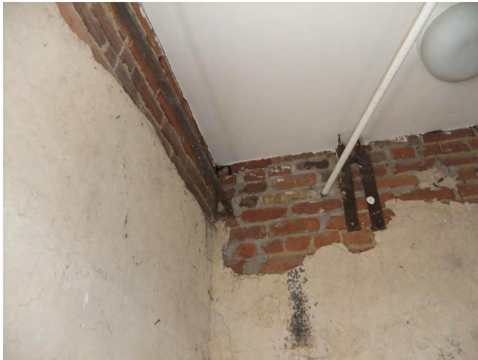
Figure 14: Attic level tie rods at northwest corner of mill
