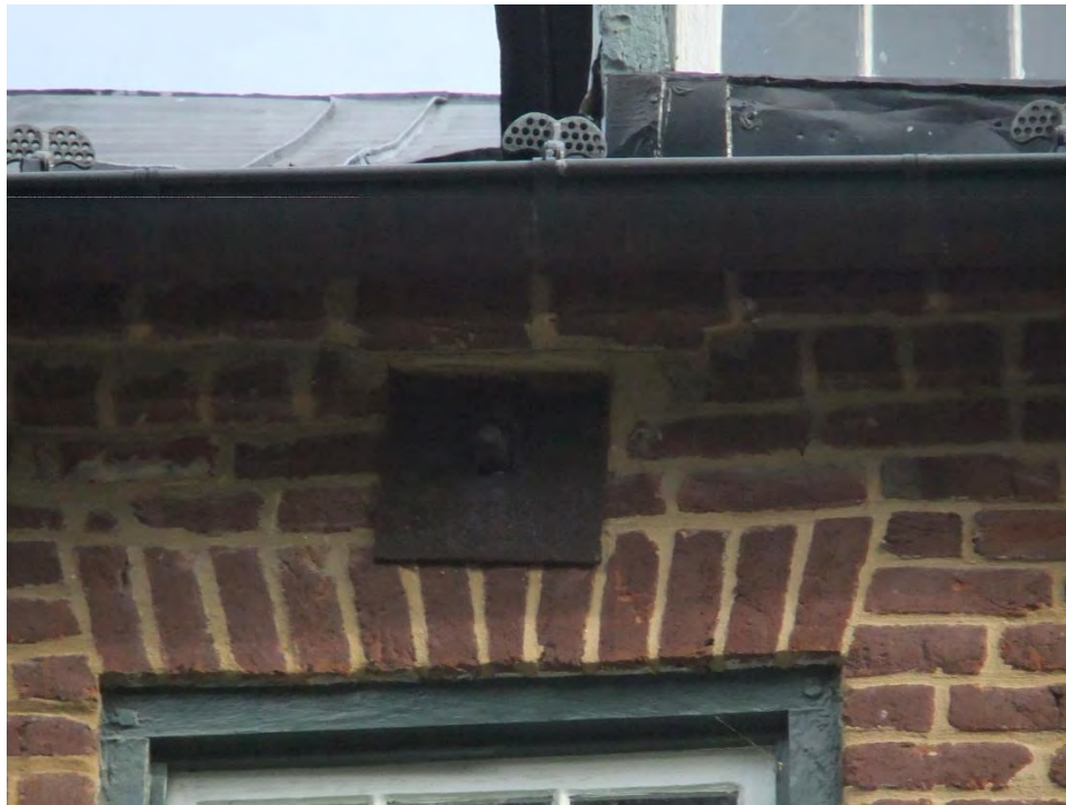
Figure 54: 20 th century tie rod anchorage below attic level
