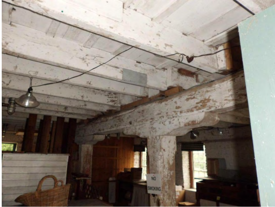
Figure 23: Second floor joist and leveling shims
