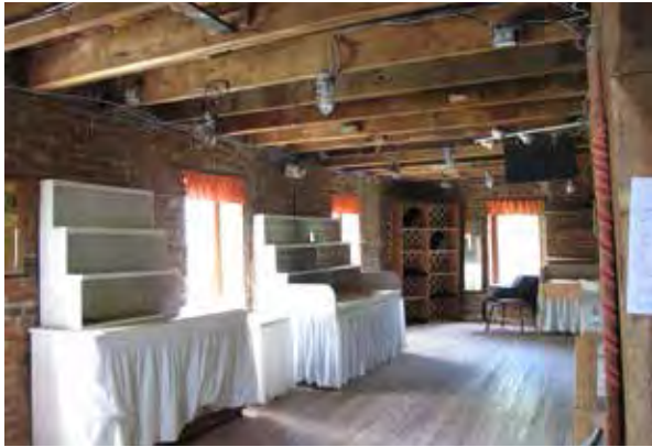
South bay of the second floor looking west.
