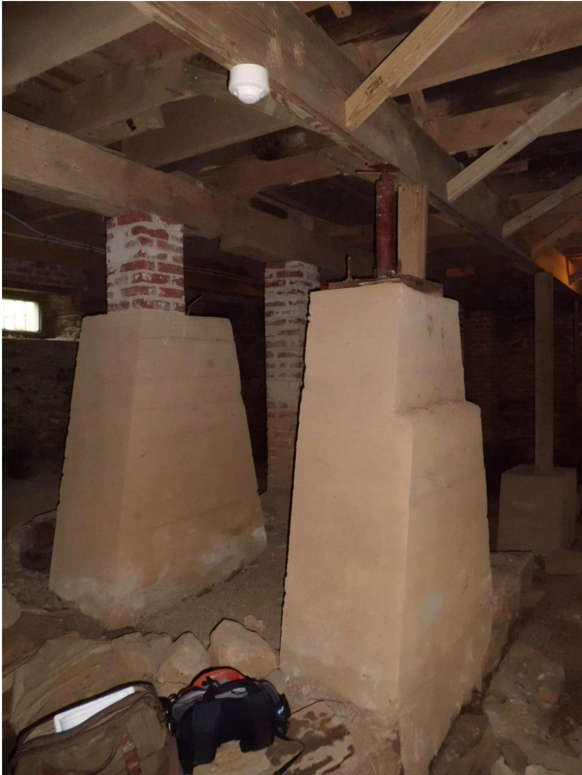
Figure 34: First floor shoring and new masonry pier support
