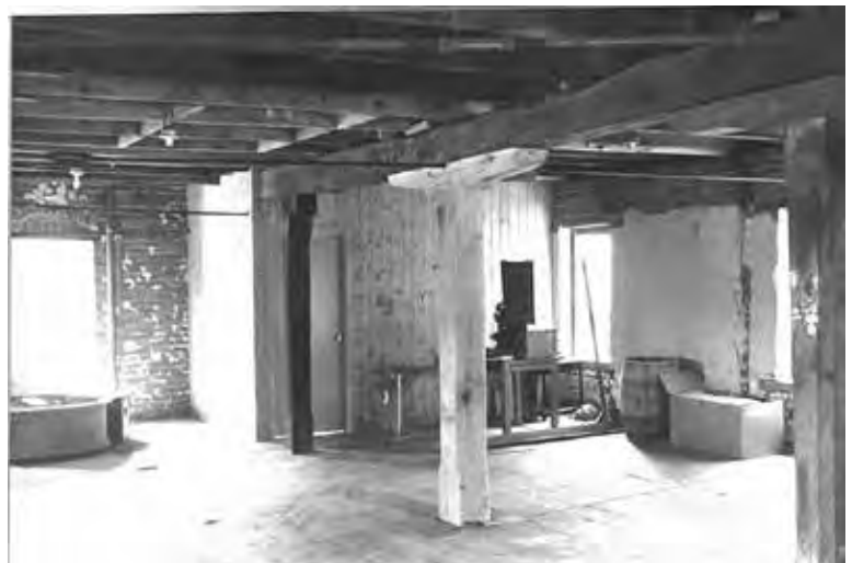
Exterior and Interior work performed in 1984 [WF].
