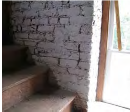
Infilled mortise for landing support at center, first-floor stair.
