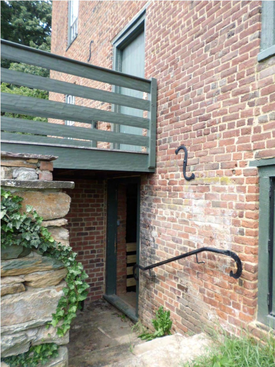
Figure 50: Installation of new first floor and basement entry along west wall
