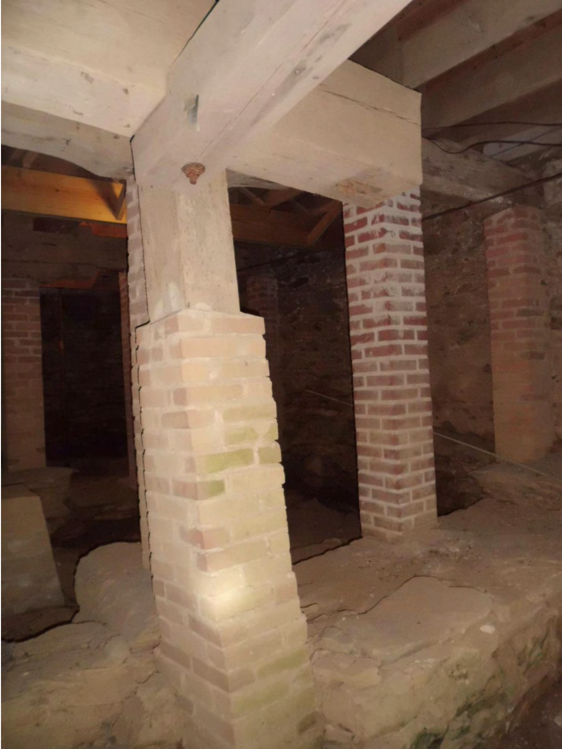
Figure 40: First floor canted brace masonry pier support
