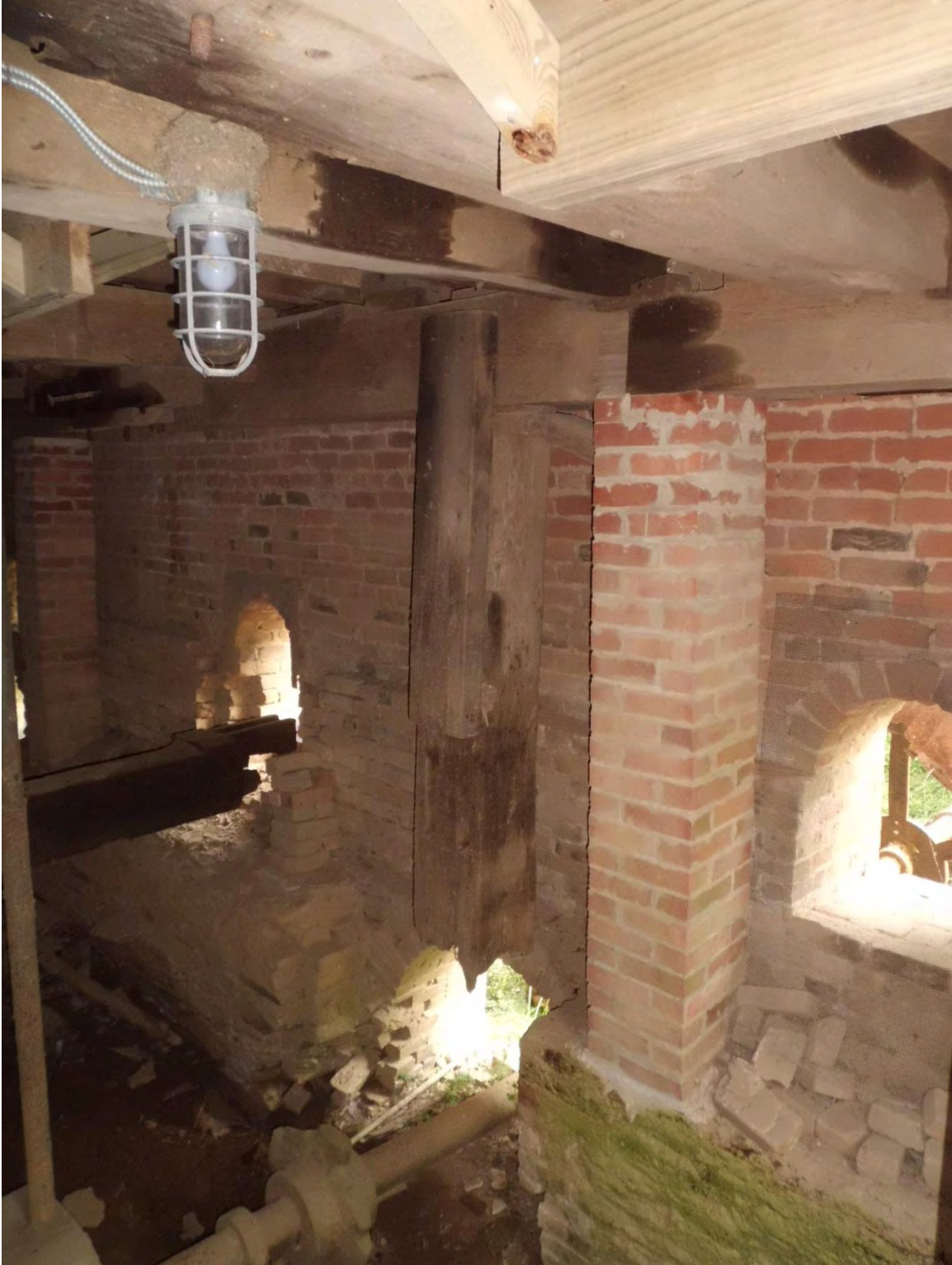
Figure 39: First floor joist supported on Hurst frame
