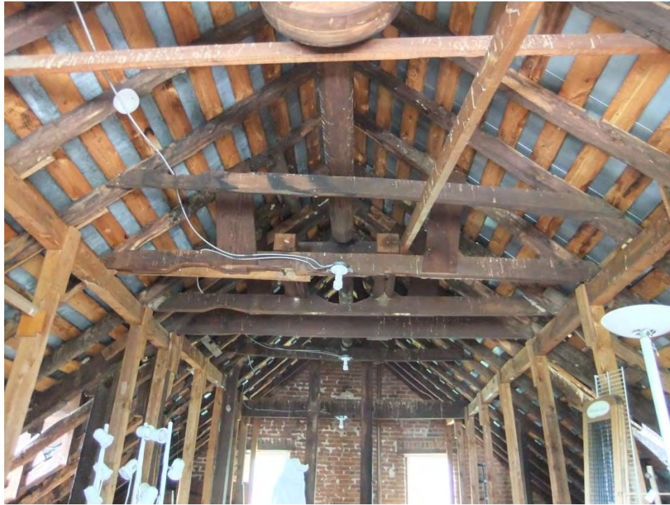
Figure 3: Roof framing with rafters, collars and purlins on stud posts.
