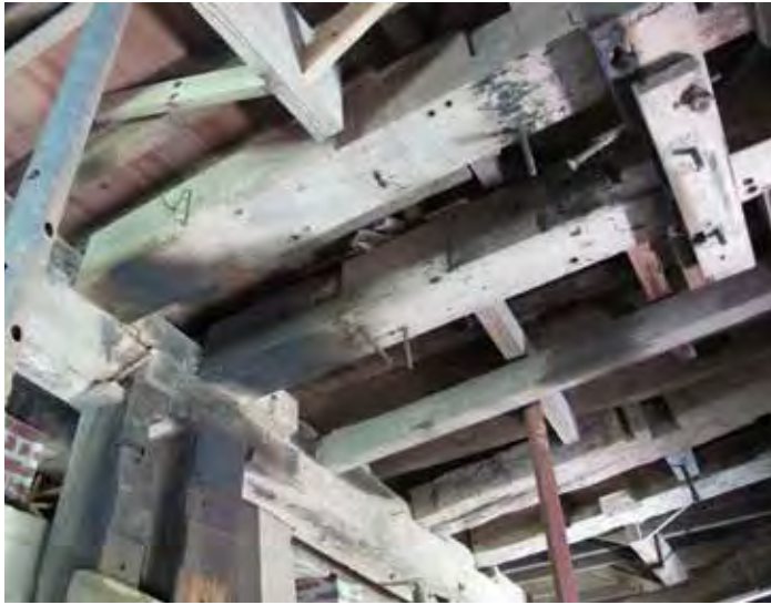
Above: Mill beam and western and central stone bearers looking northeast.
