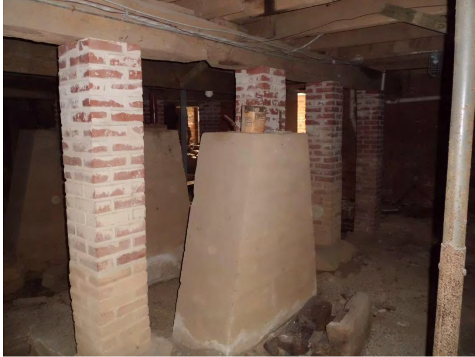
Figure 33: First floor beam re-supported on new masonry piers
