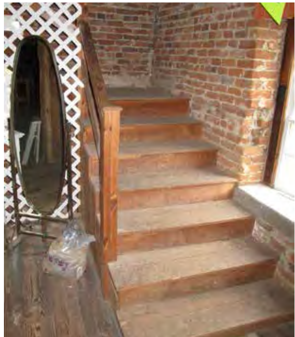
Above: The second-floor stairway showing modern risers and treads. The earlier landing may have been supported on a joist that was held in the notch in the window jamb just above the sill before the stair turned and descended to the north.
