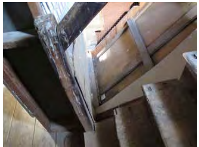
Stair to attic showing original baluster locations, newel post and rail.
