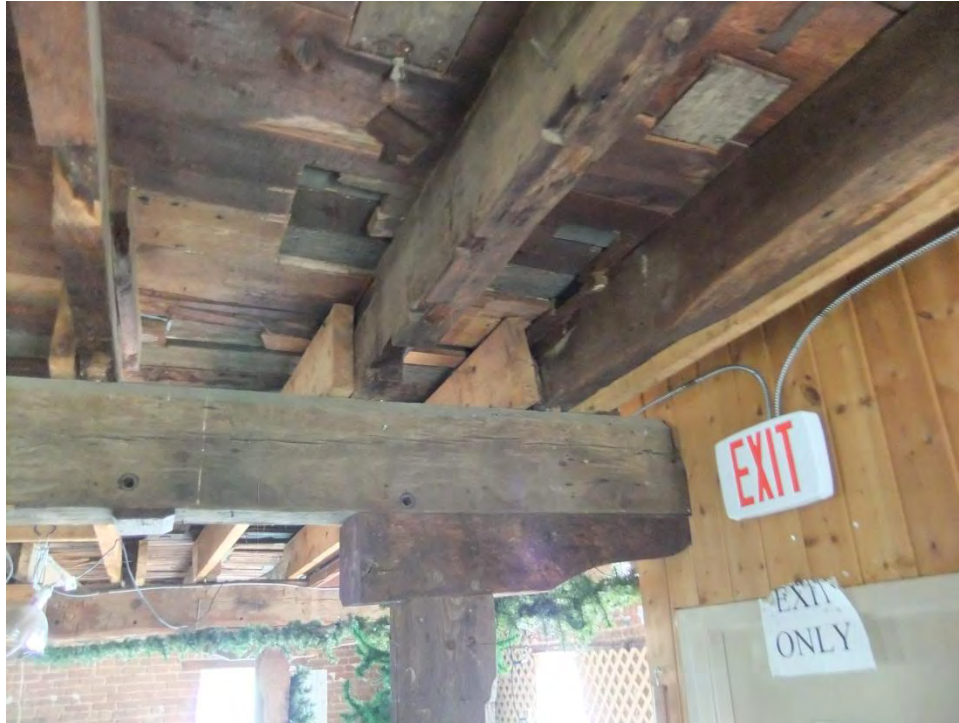
Figure 15: Attic floor framing modifications
