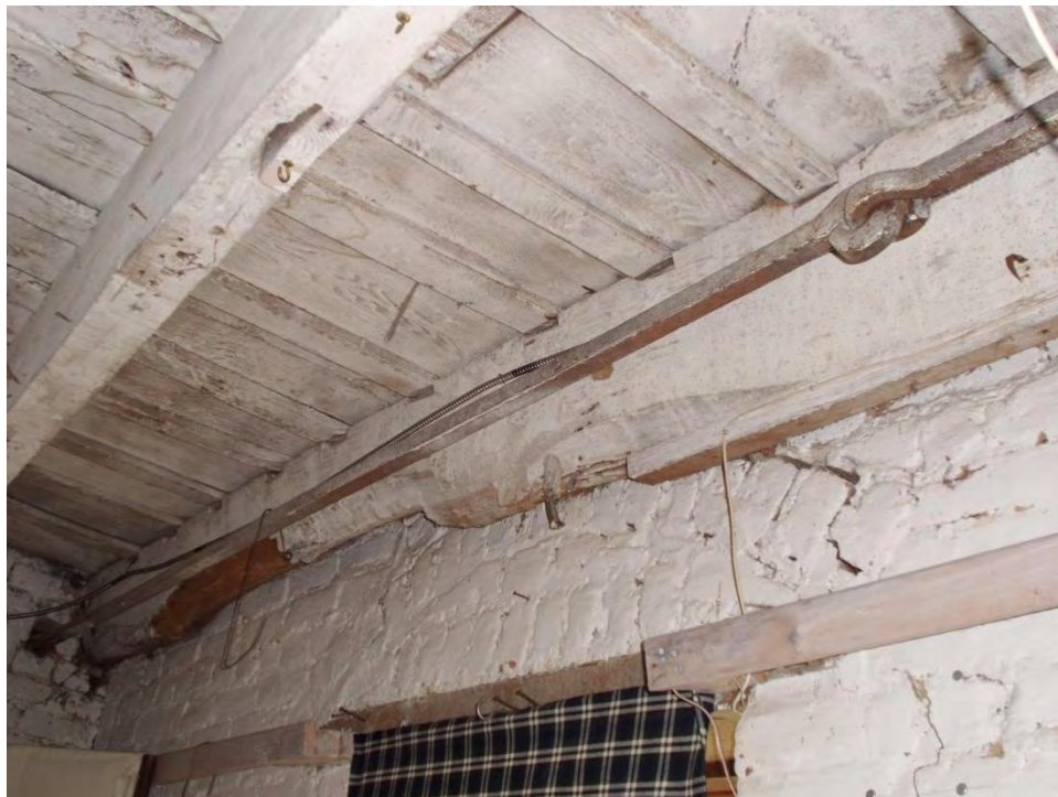
Figure 22: Tie rod at west gable wall
