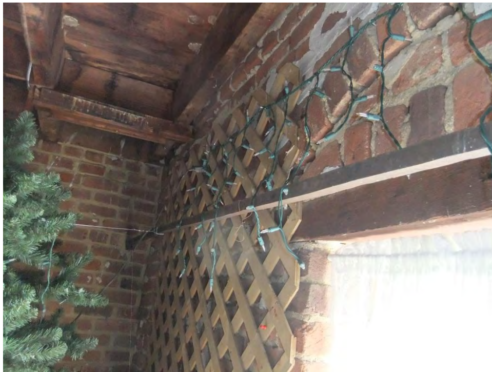
Figure 12: Attic level square tie rod along west gable end
