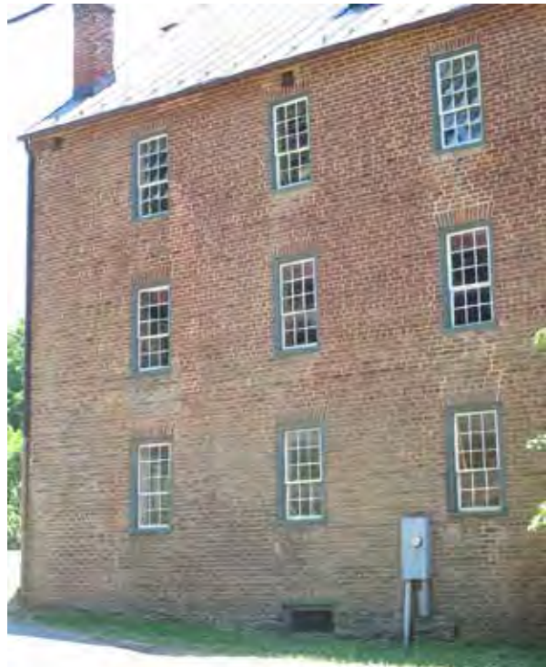
North side, Waterford Mill, 2012
