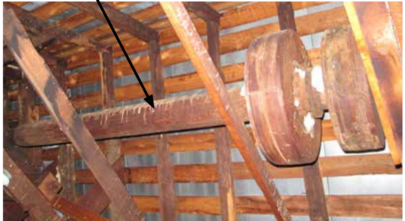
The auxiliary drive shaft and common rafters looking northwest.
