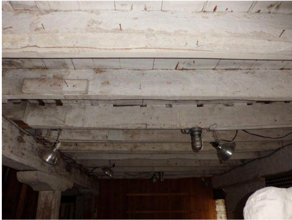
Figure 21: Second floor joist framing
